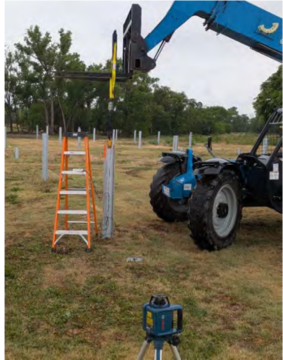
Calibrated up (extraction) pressure test:
