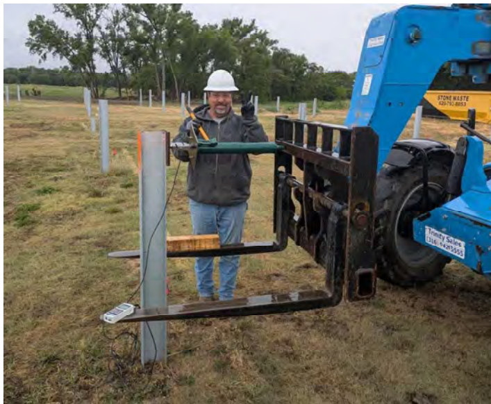
Calibrated lateral bearing test setup:
