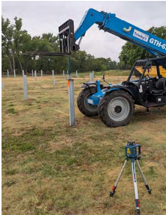
Calibrated down (bearing) pressure test
