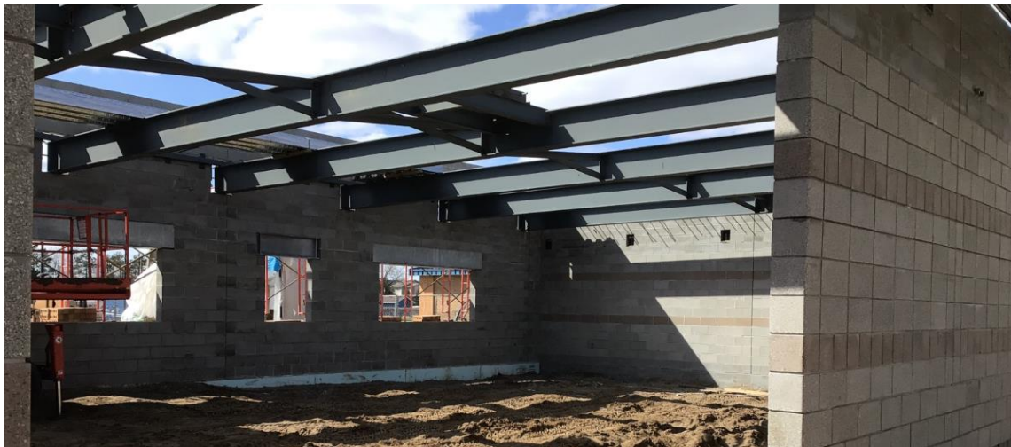
South Addition ready for decking
