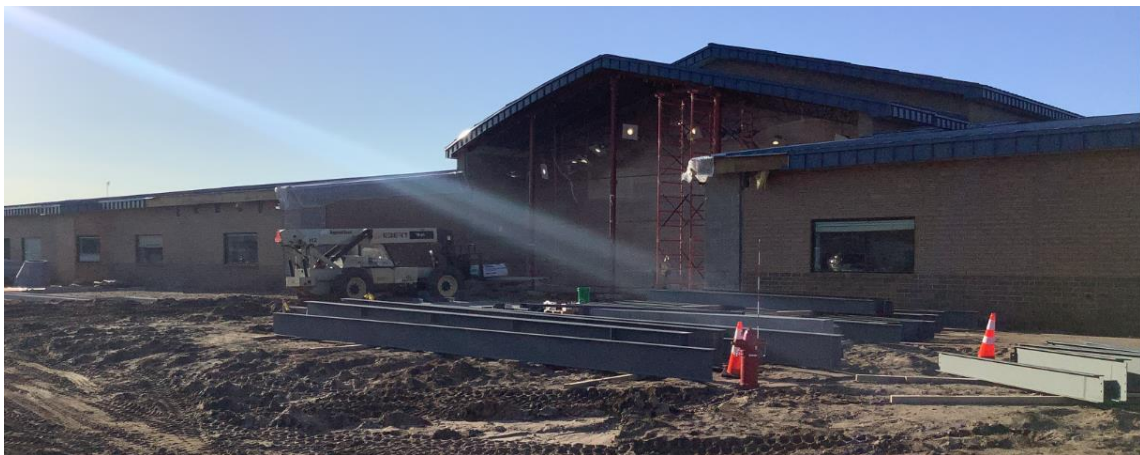
North Addition steel to begin.
