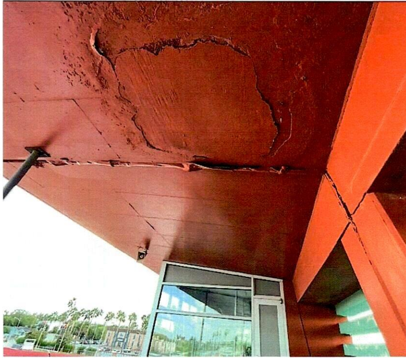
Photo 7: Patch of Roof Slab Underside due to Removal of Light Pole. Patch is Suspect to poor Adhesion and Posing a Potential Hazard of Becoming Falling Debris.
