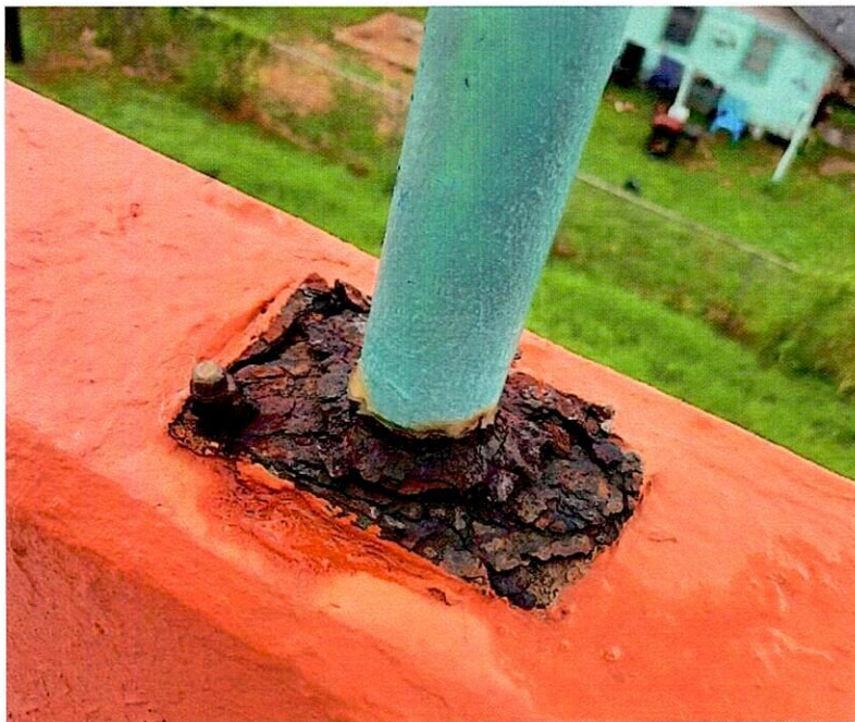
Photo 8: Guard Rail Base Plate showing Severe Corrosion.
