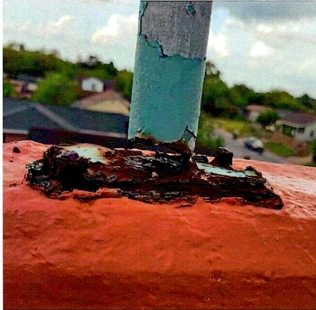
Photo 9: Guard Rail Base Plate Showing Severe Corrosion.
