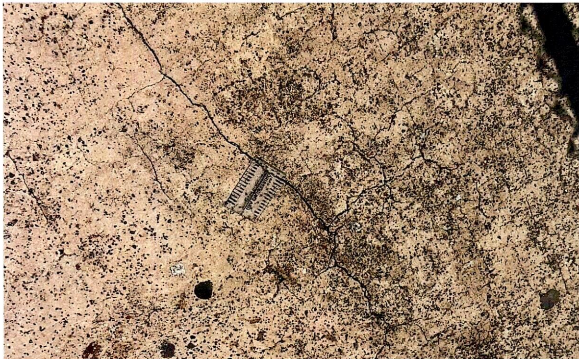
Photo 12: Shrinkage Cracking on Slabs.
