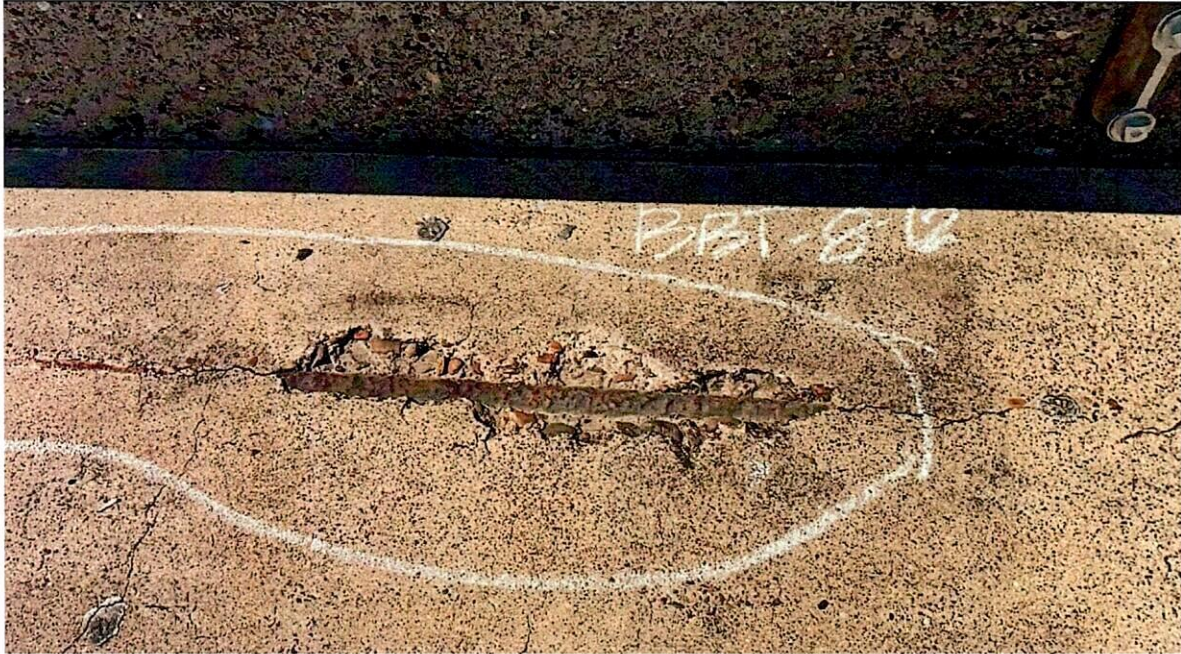
Photo 11: Bleacher Beam Topside Showing Exposed Rebar.
