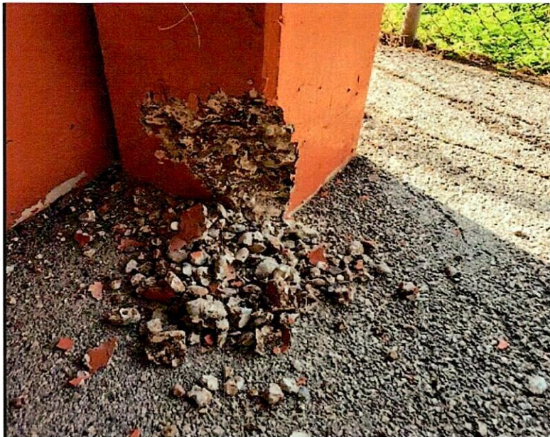
Photo #2: Column is Experiencing Spalled Concrete.
