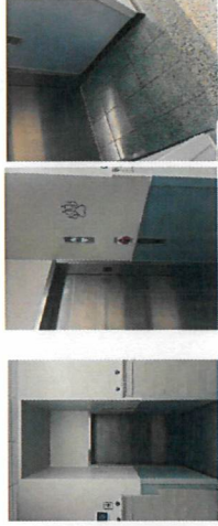
EXISTING CONDITIONS PHOTOS - THIRD FLOOR
