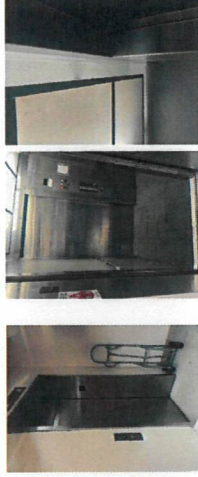
EXISTING CONDITIONS PHOTOS - LOWER LEVEL
