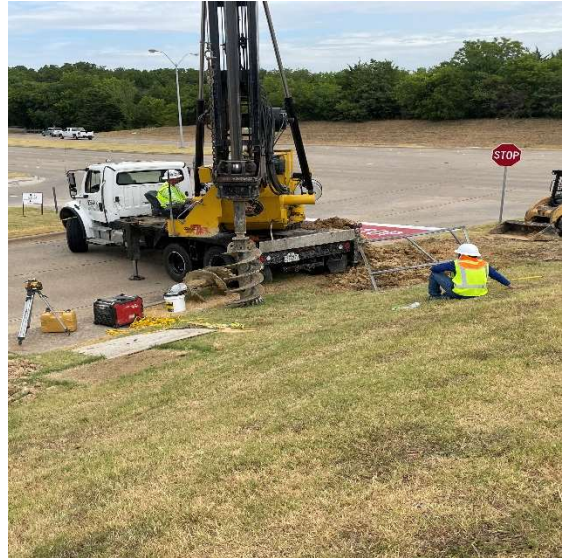
Drilling Piers at Spring Creek Sign
