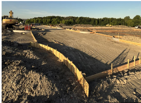
Forming Fire Lane
