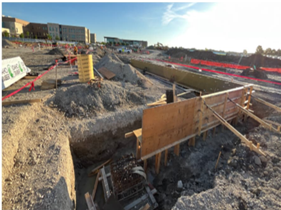
Forming Grade Beams
