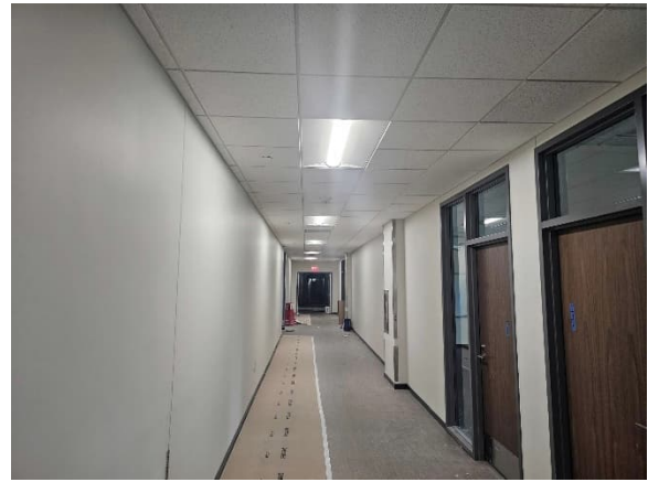
E Wing 1st Floor Hallway
