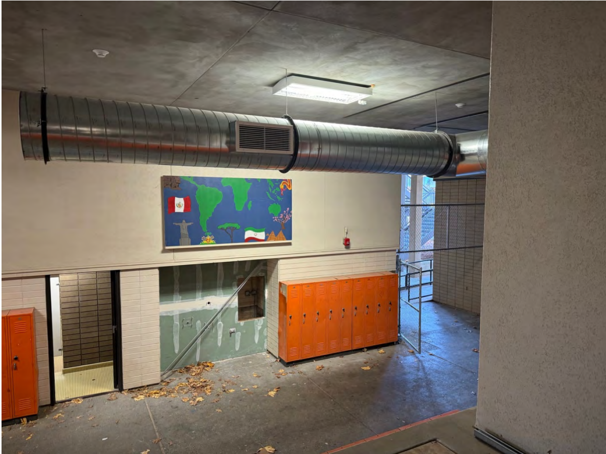
AHS Tech Level Improvements in Progress
