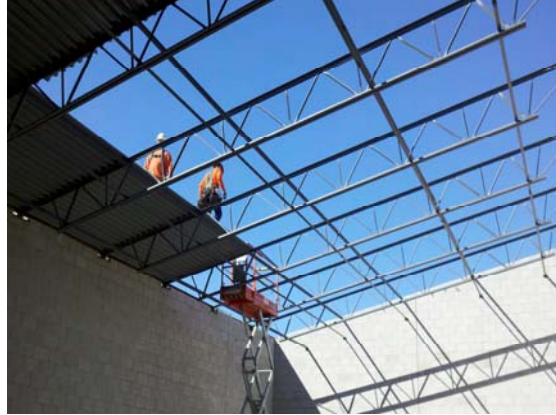
Roof Framing and Decking Installation
