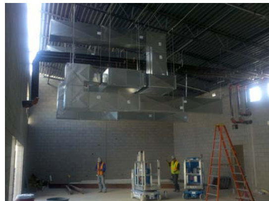
Mechanical Equipment Installation
