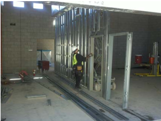
Interior Wall Framing
