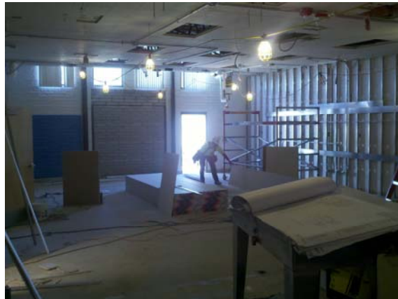
Remodel of old comp lab into new choir room
