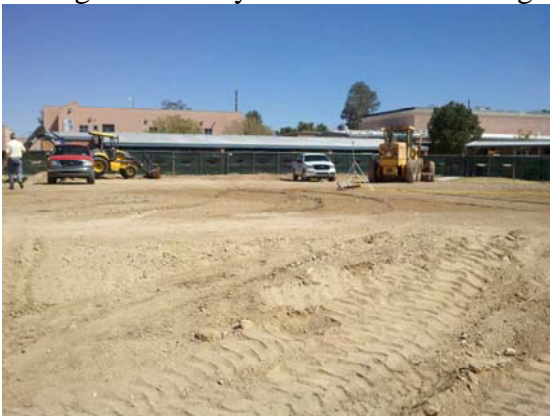
Building Pad Prep
