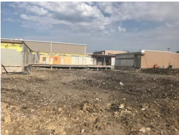
Area A Debris Haul-off/Clearing
