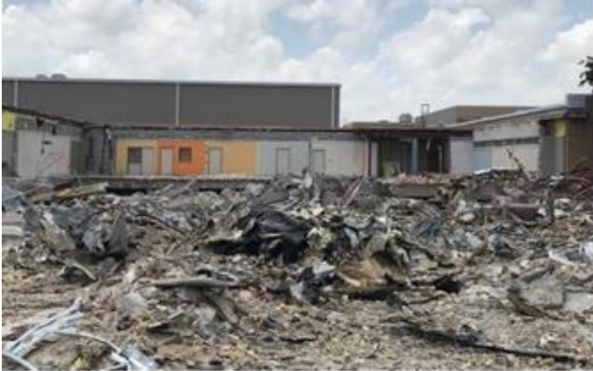
Area A Demolition
