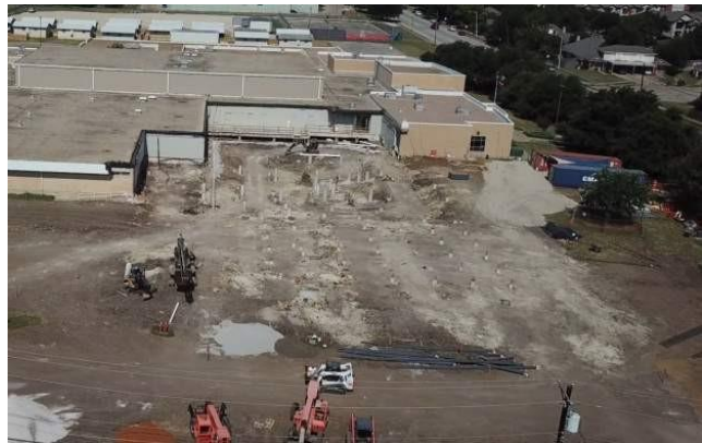
Area A Piers
