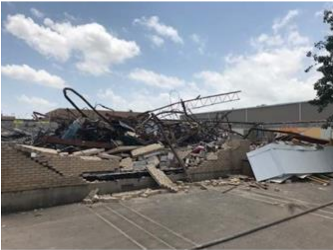
Northwest Corner Area A Demolition
