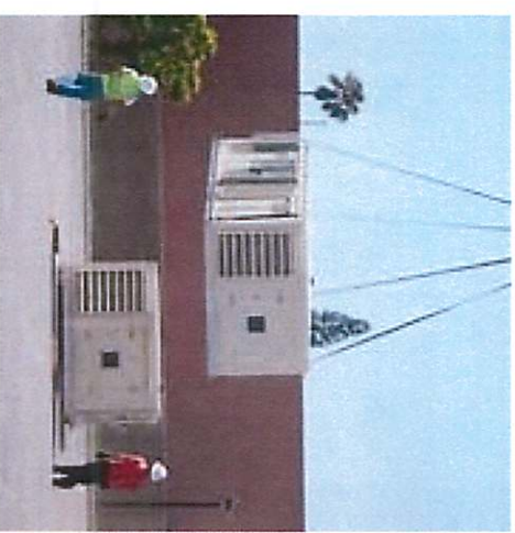
RTU's Past the End of their Useful Life Replaced
