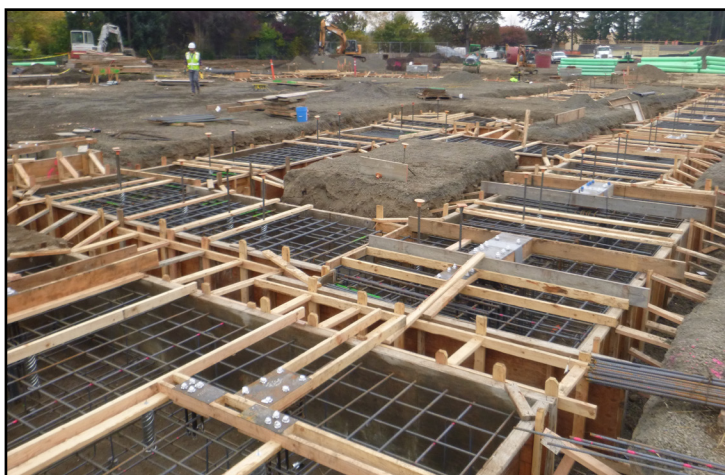
Footing forms and rebar in gym
