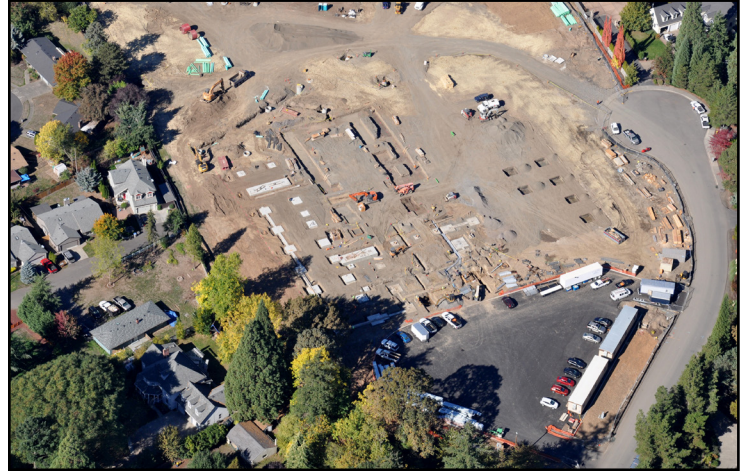
Aerial view looking Northwest
