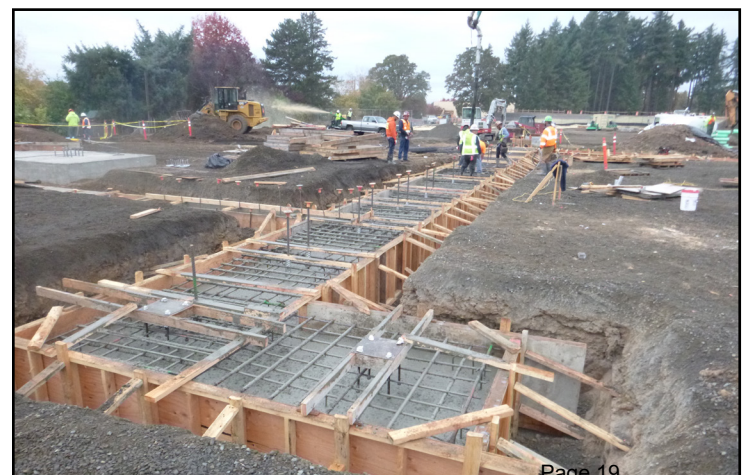
Concrete placed in strip footing under gym wall
