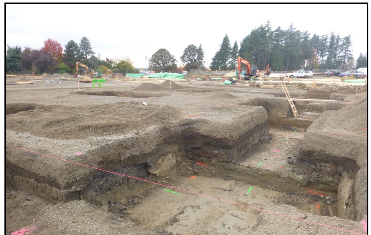
Footing excavation in kindergarten area
