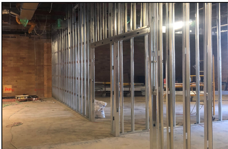
Northeast stud walls
