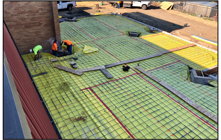
Concrete slab preparation
