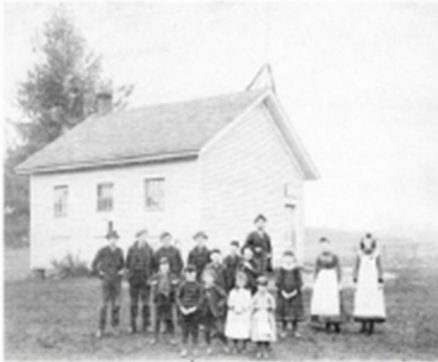
Public school at NE 122 nd and Sandy, Parkrose, ca. 1890. OHS photograph.
