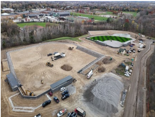
Aerial View Earthwork
