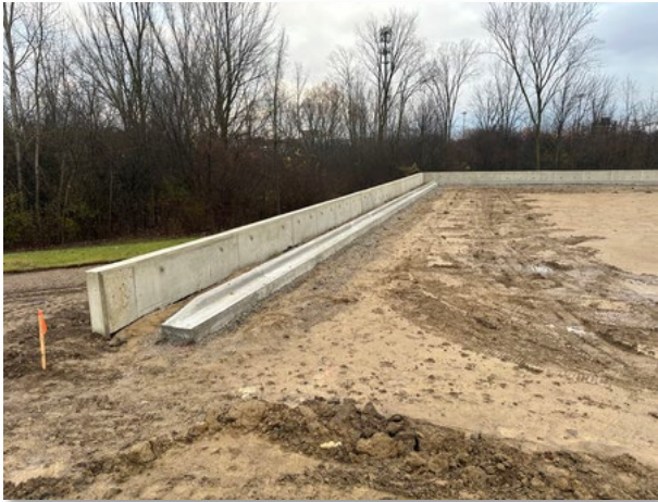
Parking Retaining Wall
