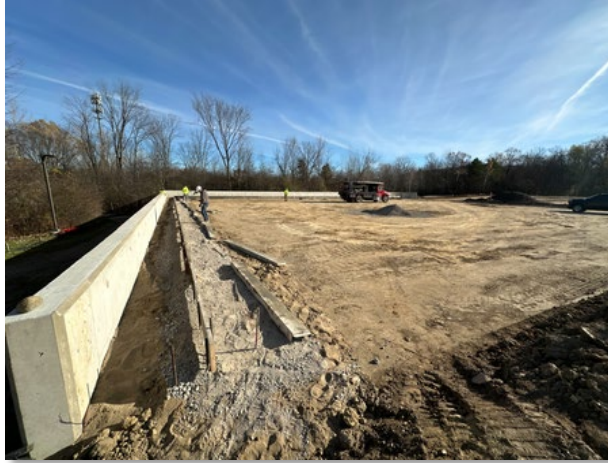
Concrete Retaining Walls
