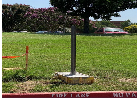
Tube and Foundation for Wayfinding Signage
