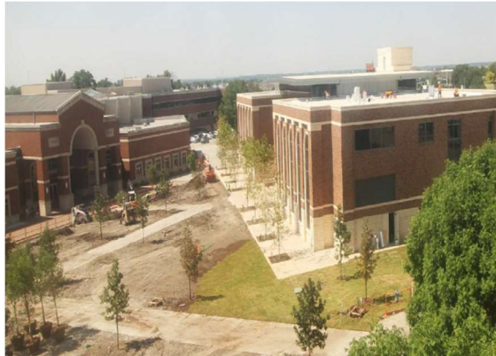
Sidewalks and Colored Concrete Poured
