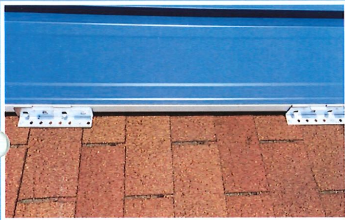
Clip seated on two shingles with fasteners through lower ends of the shingles.
