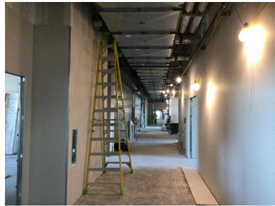
Second Floor Hall in North Building
