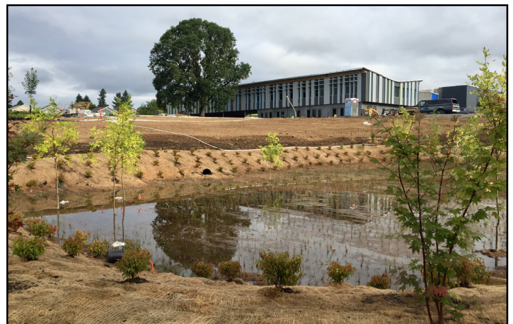
Storm water pond
