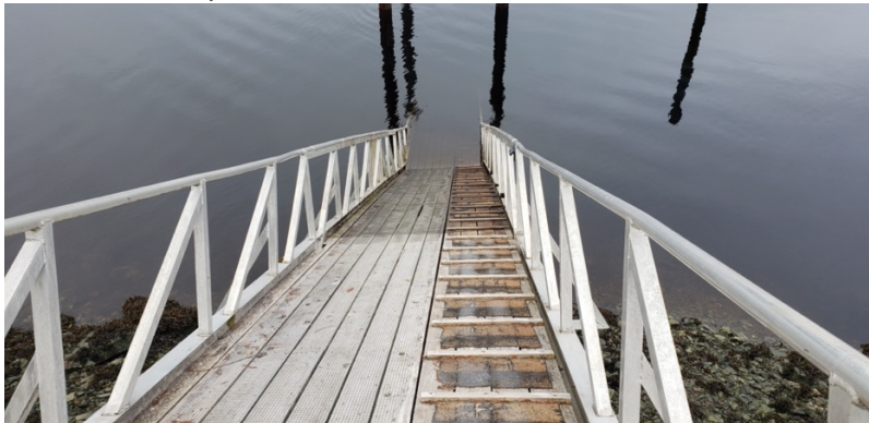
Picture of Ramp
