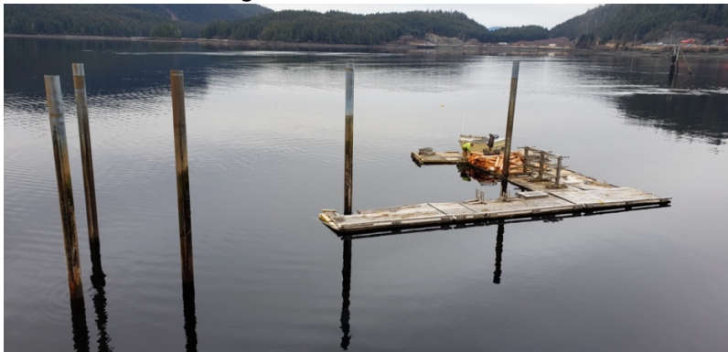
Picture of Metal Pilings and Dock Parts
