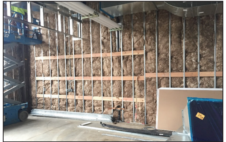
Classroom insulation and backing
