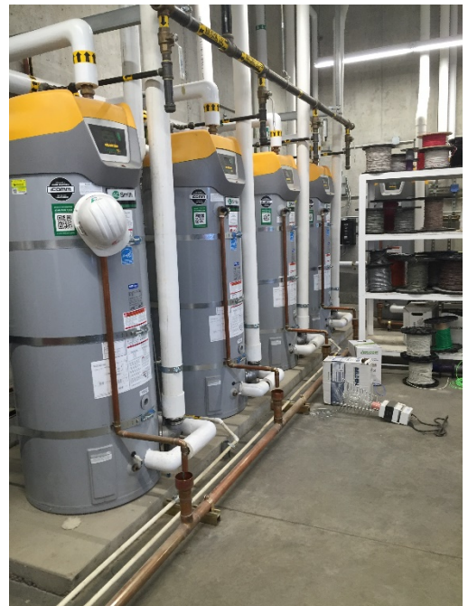
Condensing Hot Water Heaters
