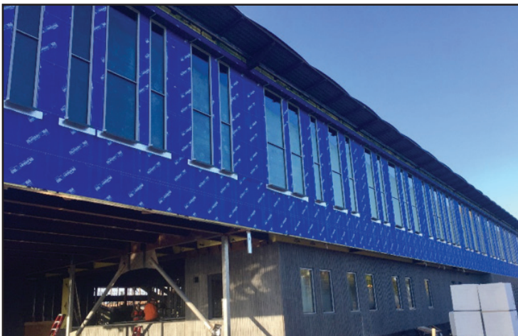
Windows at entry
