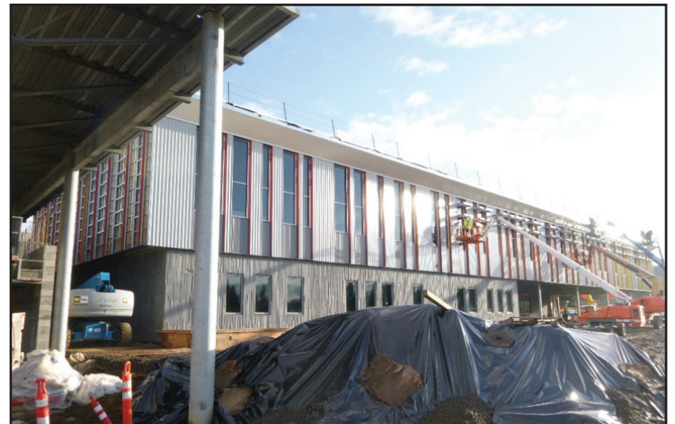
Exterior metal paneling
