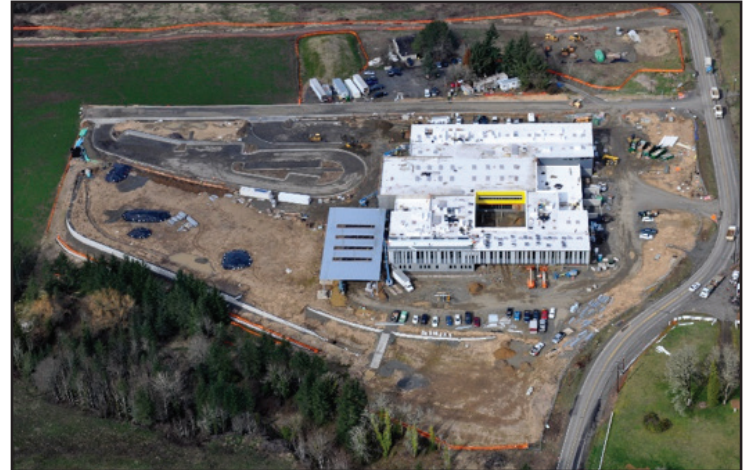
Aerial looking north
