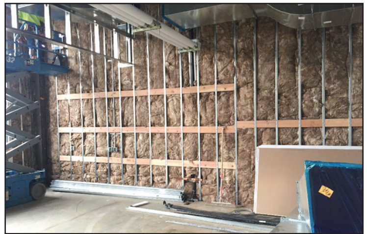
Classroom insulation and backing
