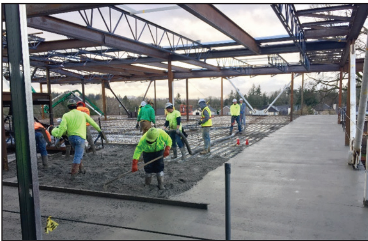
2nd floor classroom concrete pour
