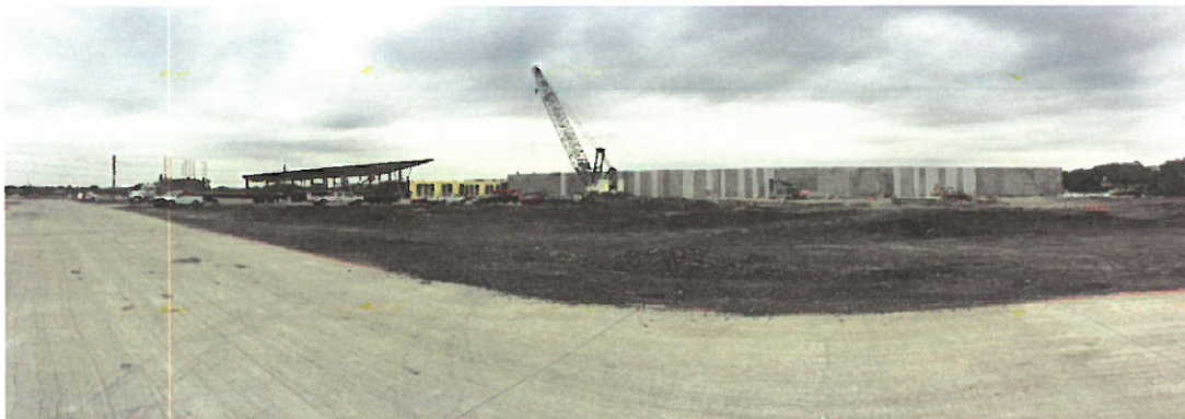
Bldgs. A,B,C & D panorama viewed from SE
