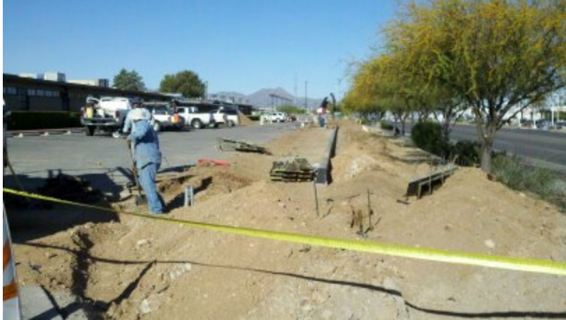
New Curb Installation for Increased Parking
