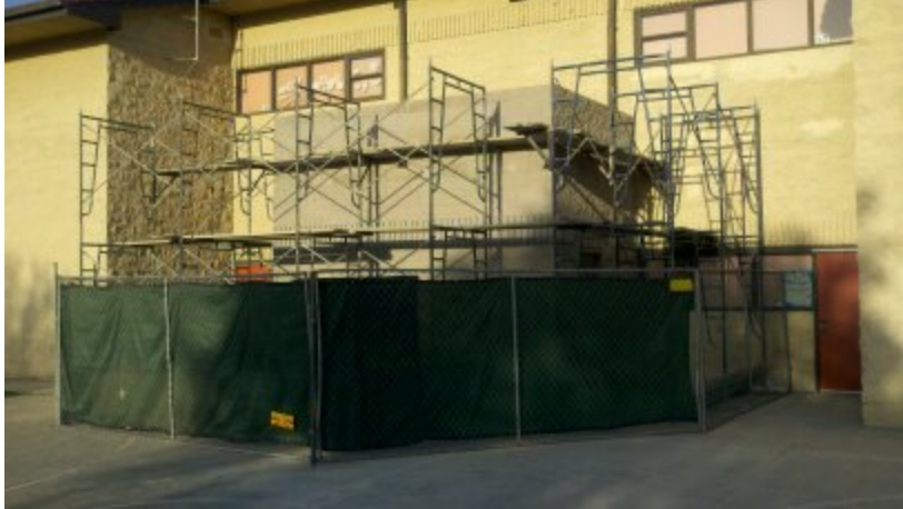
New Masonry IDF Construction
