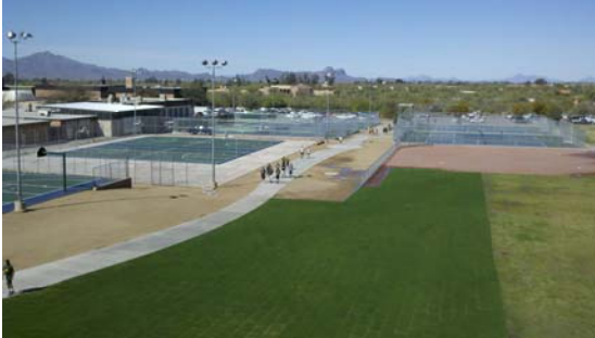
New Tennis Courts and Walkway
