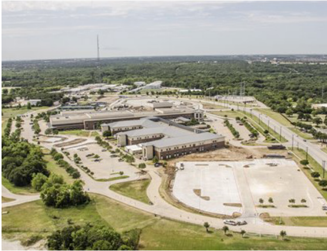
North parking lot completed
