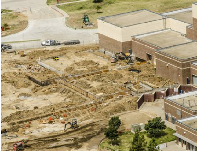
Area 'D' Grade beams in progress
