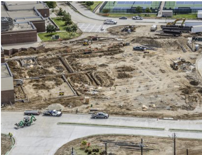
Area 'D' Grade beams
