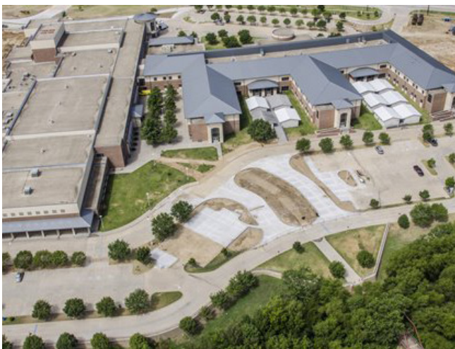
East parking lot paving in progress
