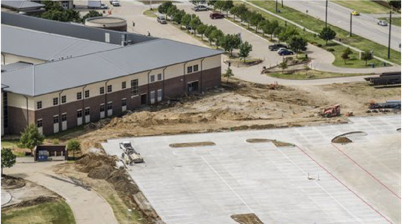
Area 'C' Piles Complete (view from North)
