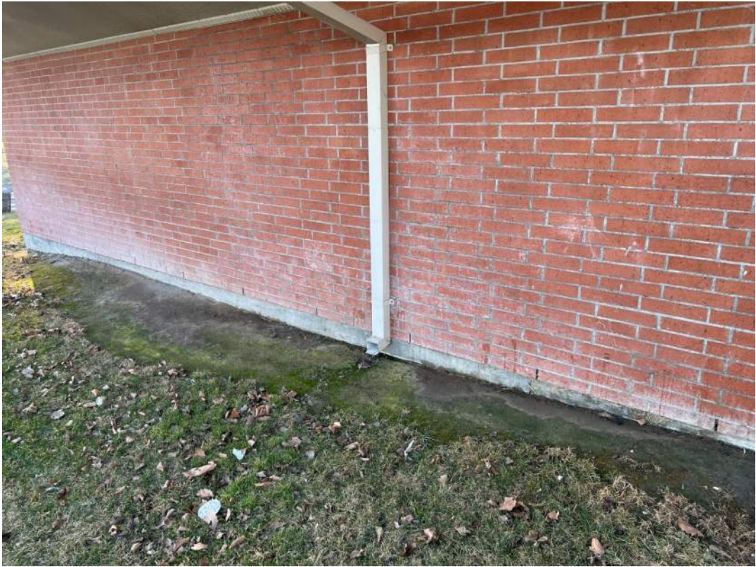
(Above: Downspout draining next to building Below: Irrigation spraying walls)
