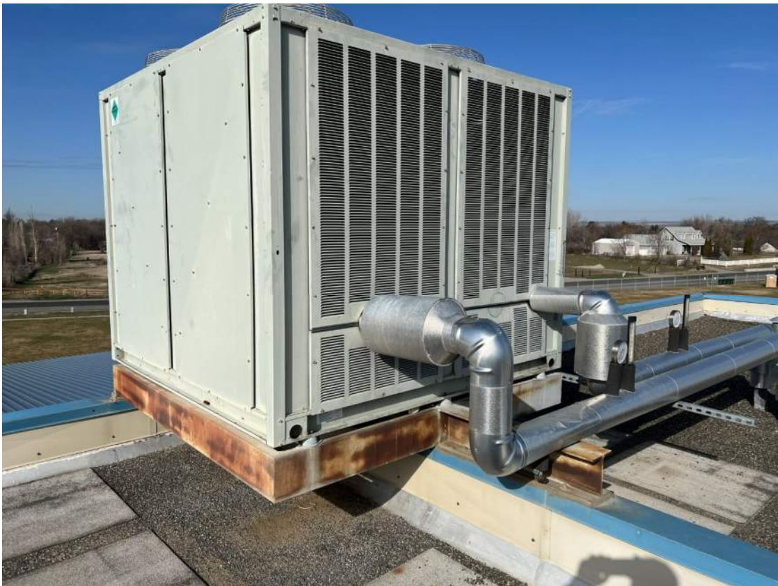
(Above/Below: Rooftop mechanical unit supported by parapet)
