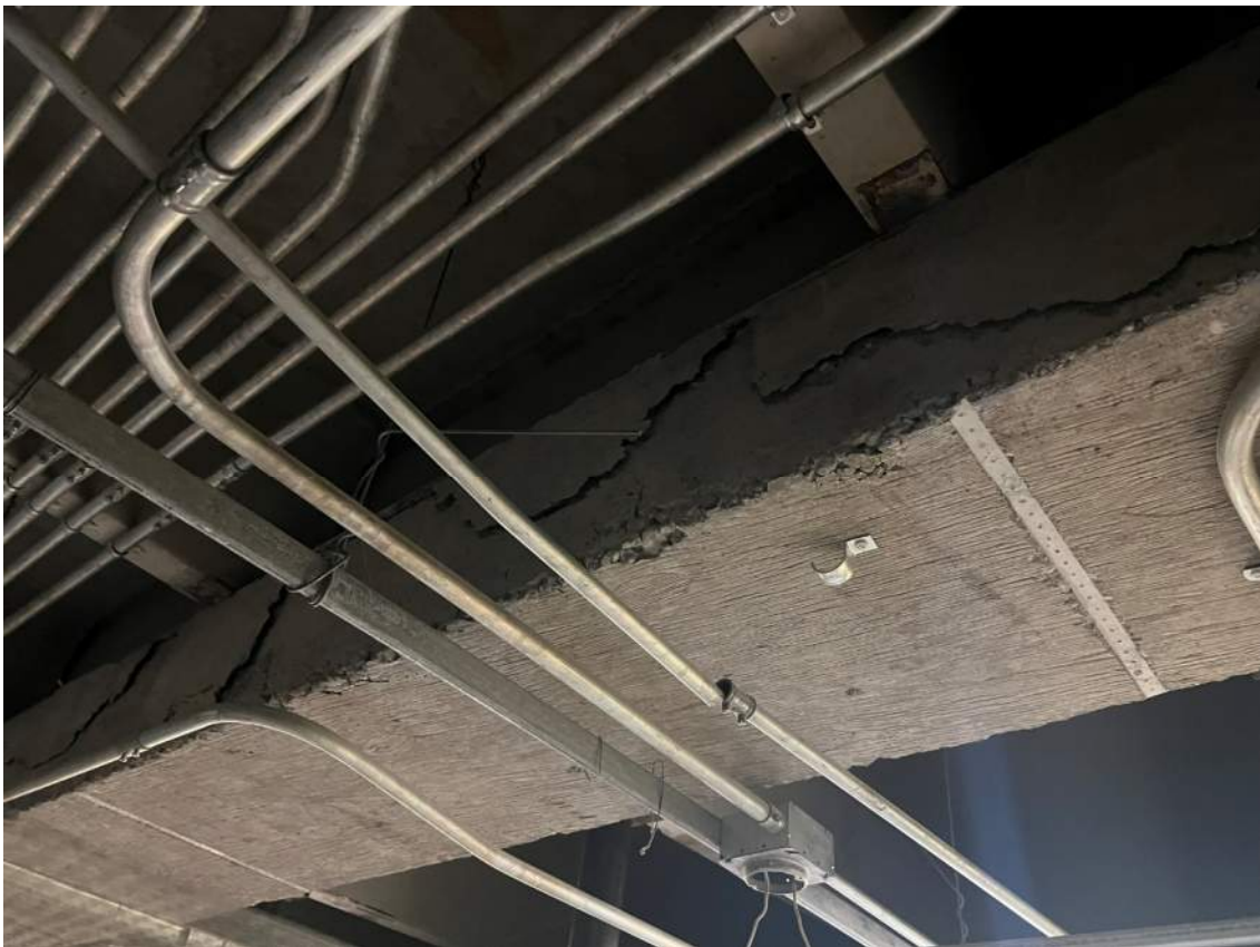
(Above/Below: Cracks in roof support beam)
