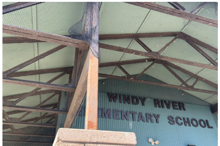
Front entry soffit
