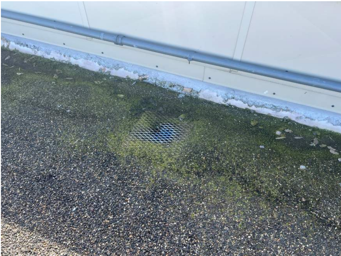
(Above: Roof drain not covered Below: Mesh roof drain cover)
