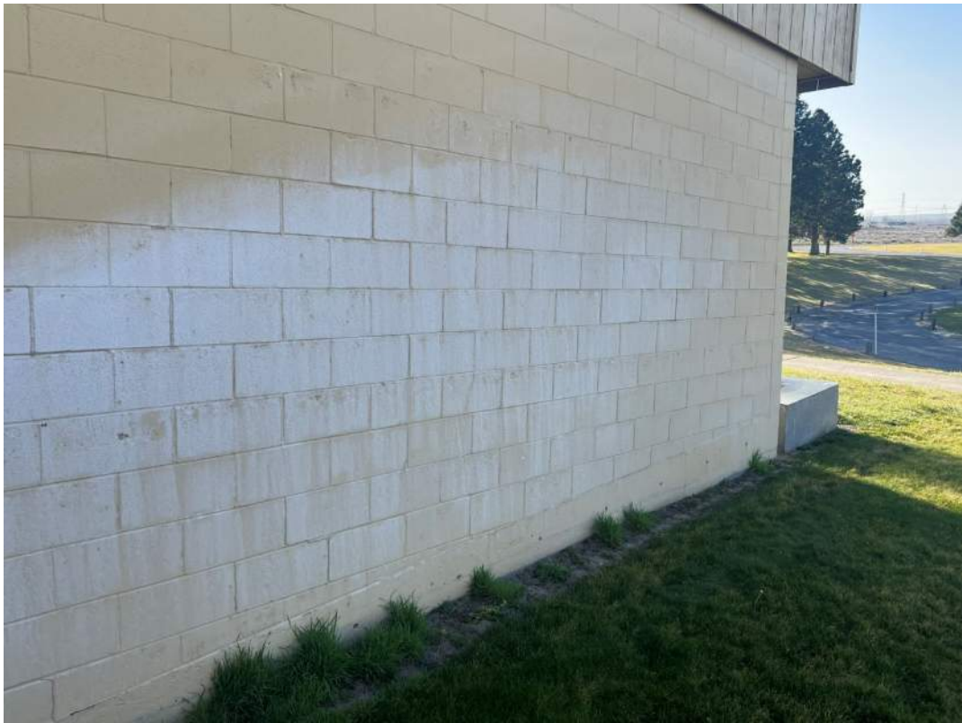
(Above: Deteriorating walls at locker rooms Below: Irrigation spraying walls)
