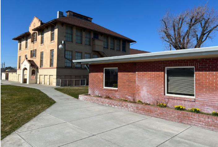
Unoccupied historic Building adjacent to school
