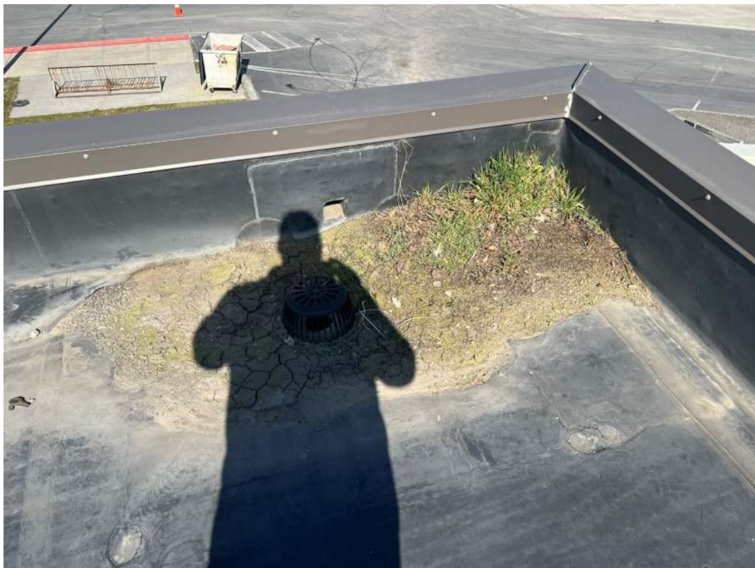
(Above: Roof debris Below: Roof debris and grass clogging drain)
