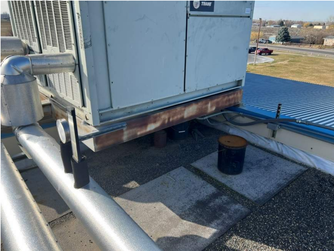
(Above/Below: Rooftop mechanical unit supported by parapet)
