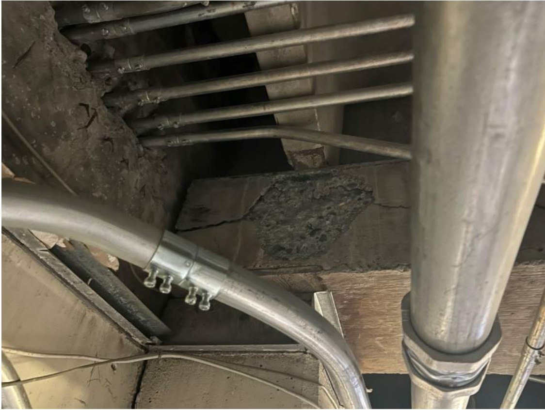
(Above: Crack/Spalling at roof support beam Below: Temporary Shoring in place)
