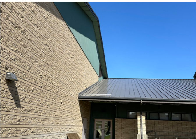
Roof and masonry
