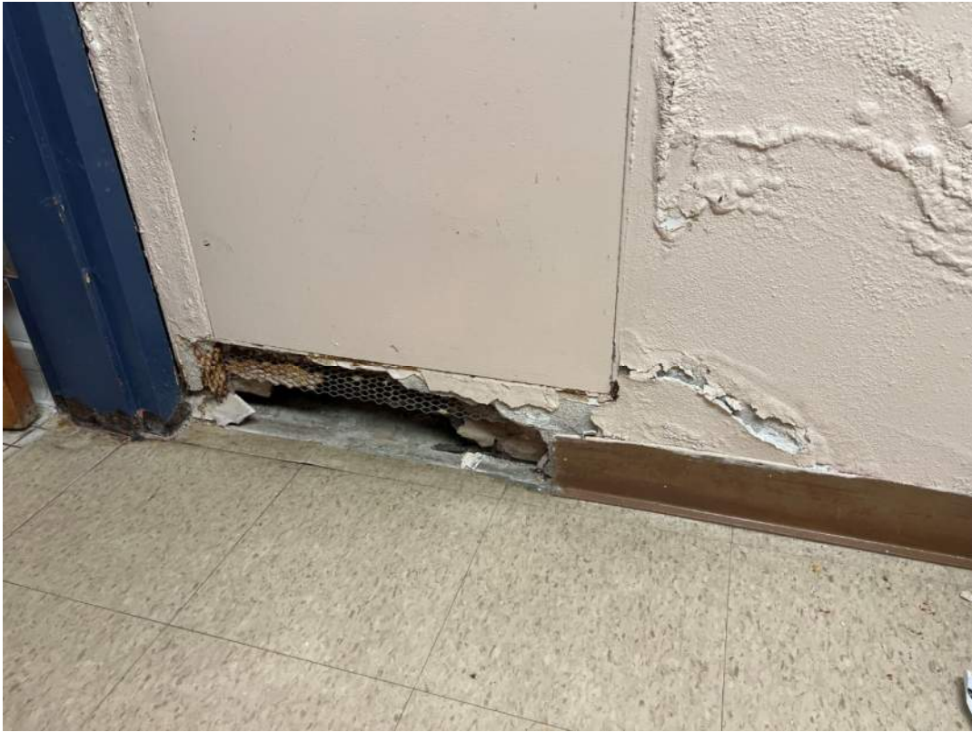
(Above: Deteriorating walls at locker rooms Below: Irrigation spraying walls)
