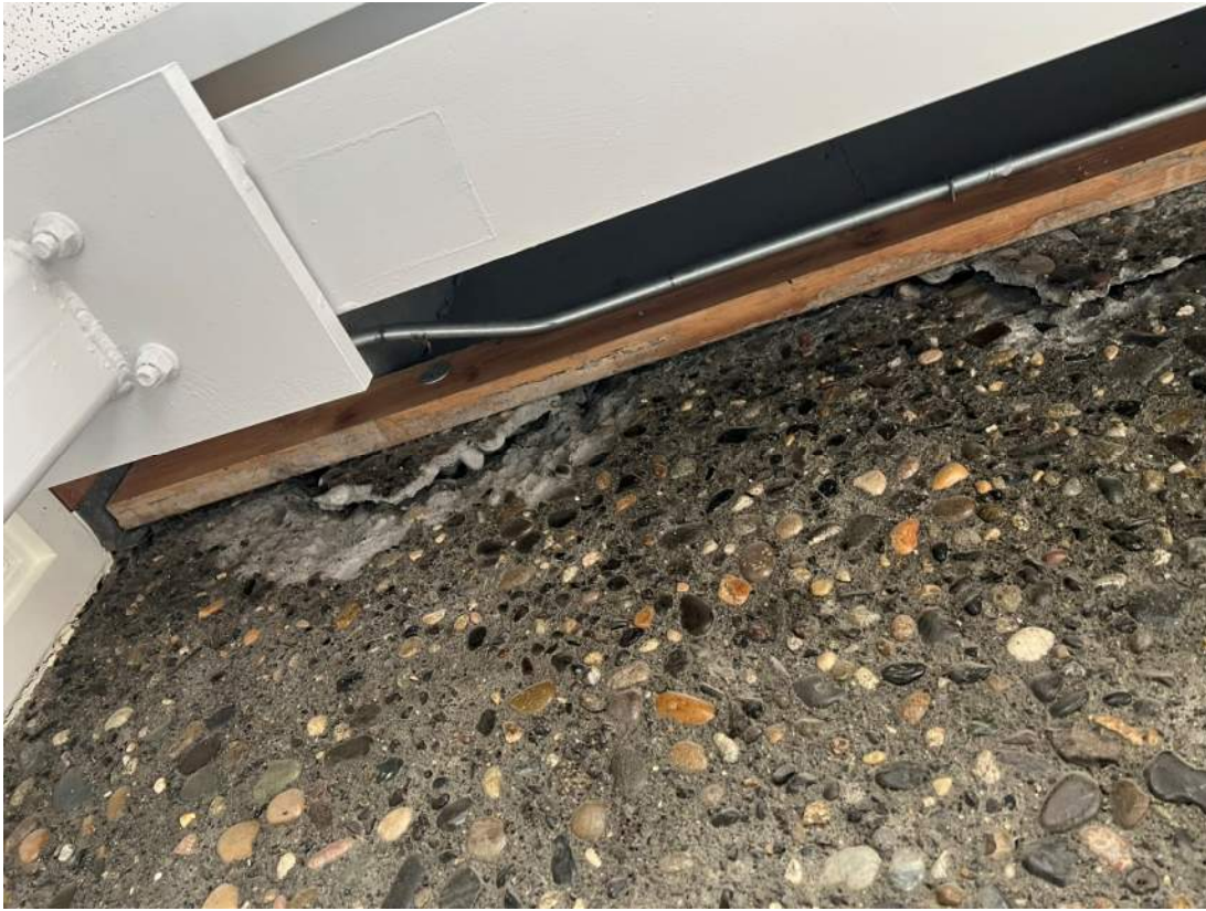
(Above: Wall Spalling Below: Cracking @ Double Tee Bearing End)
