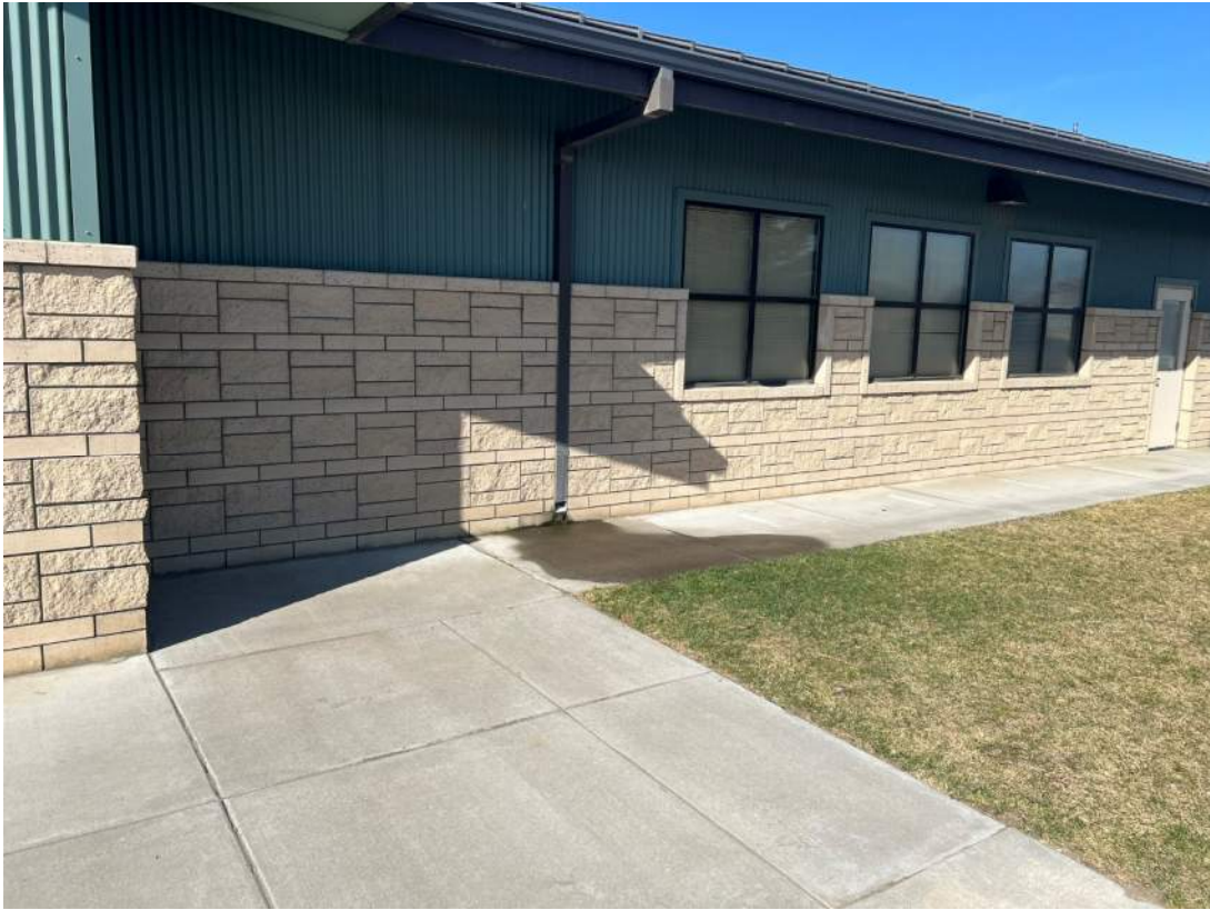
(Above: Downspout draining next to wall Below: Weathered steel @ entries)
