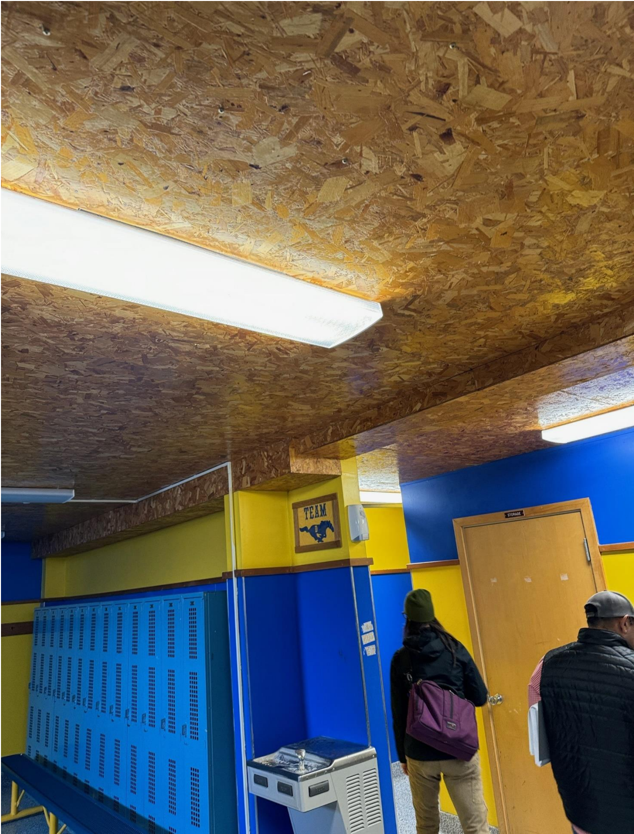
(Above: sheathing below framing for mezzanine w/ weight room above)
