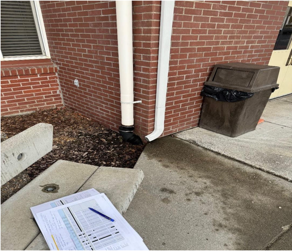
(Above: improper roof drainage at entrance
