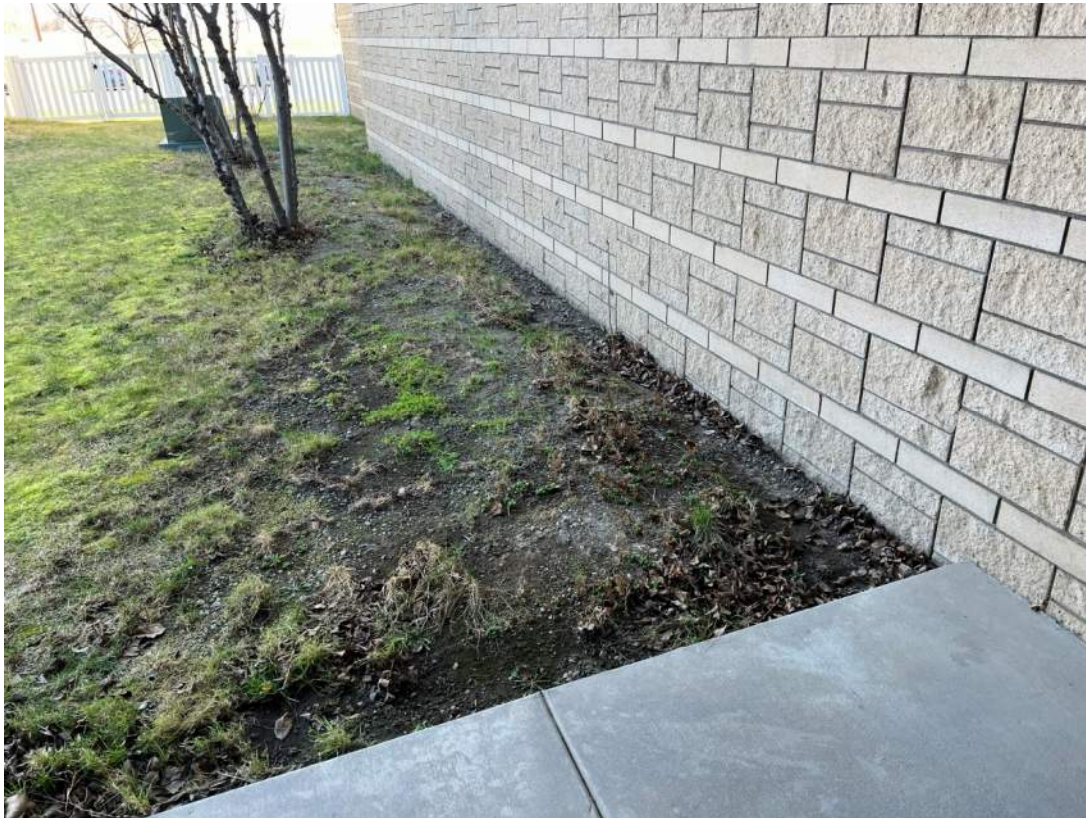
(Above: Downspout draining next to wall Below: Grade sloping toward building)
