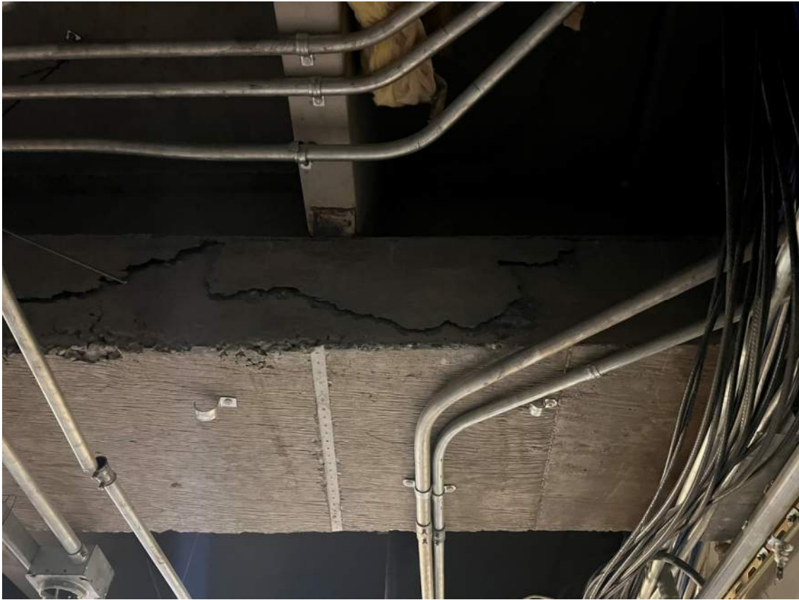
(Above/Below: Cracks in roof support beam)
