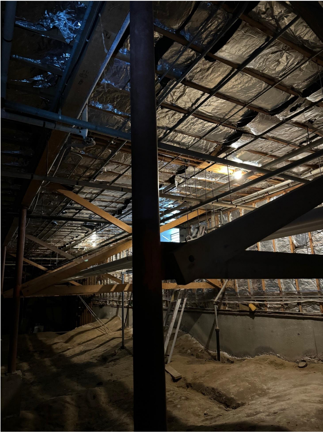
(Above: crawl space framing)
