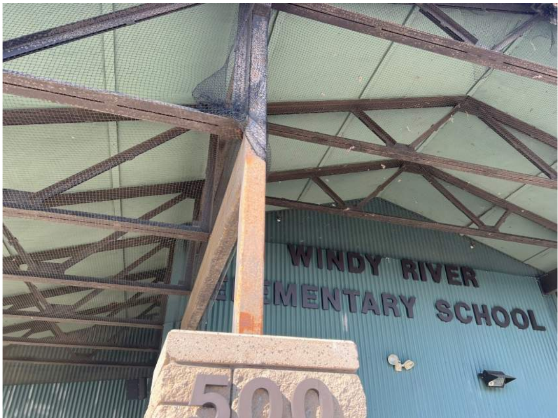
(Above: Downspout draining next to wall Below: Weathered steel @ entries)
