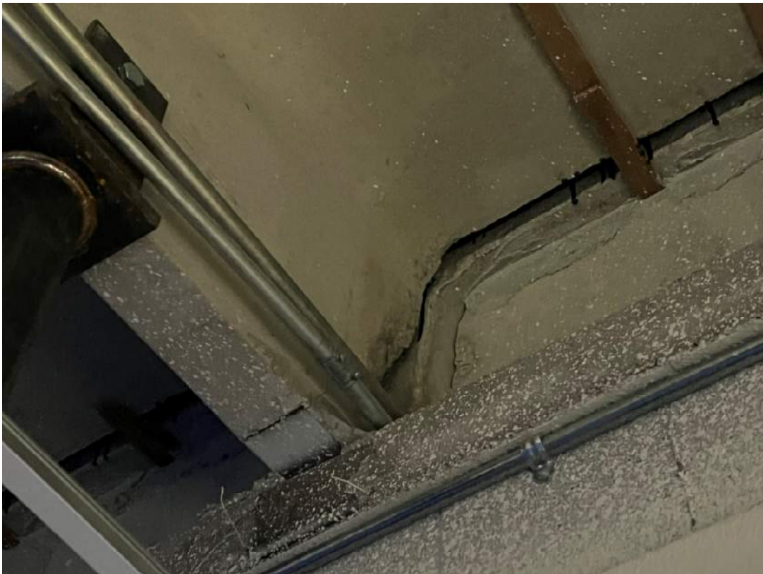
(Above: Wall Spalling Below: Cracking @ Double Tee Bearing End)
