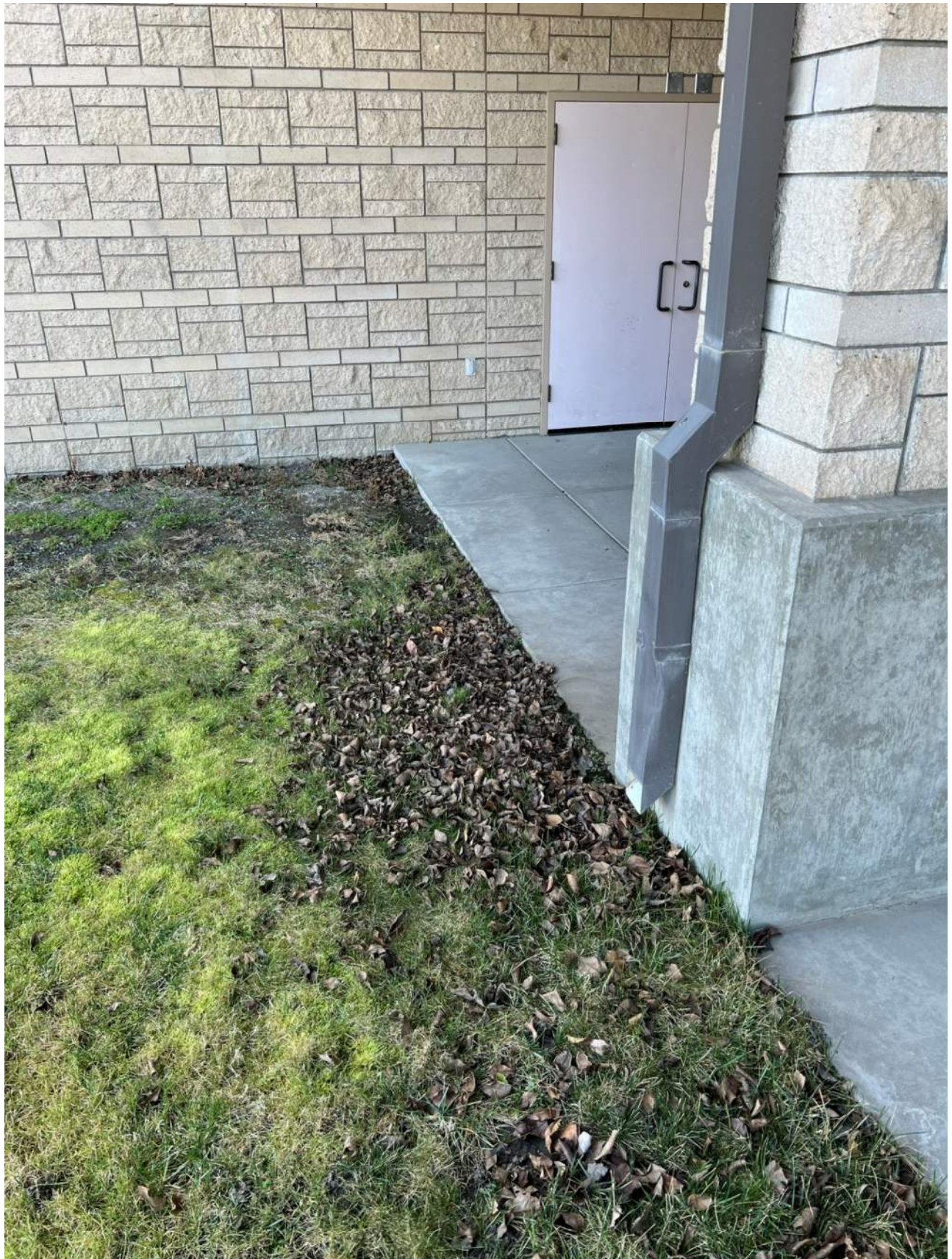
(Above: Downspout draining next to foundation and grade sloping toward building)
