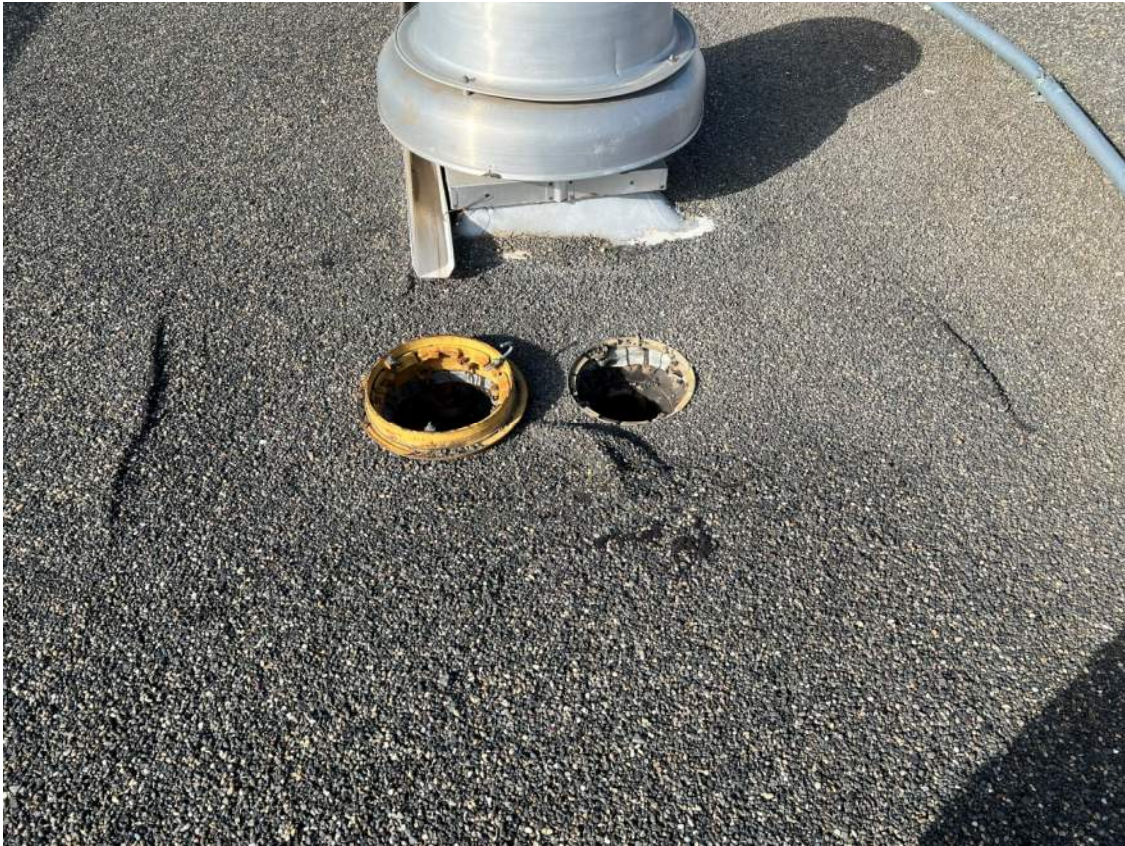
(Above: Roof drain not covered Below: Mesh roof drain cover)
