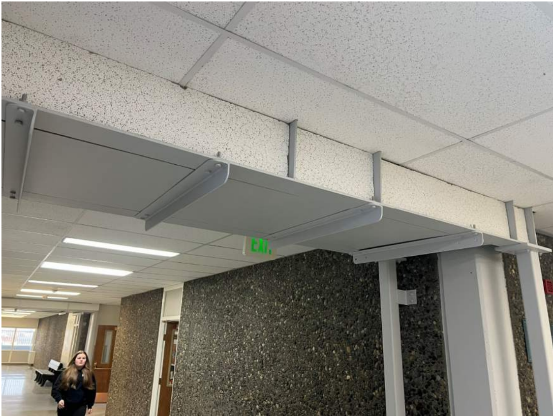
(Above: Crack/Spalling at roof support beam Below: Temporary Shoring in place)
