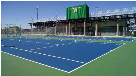
New Tennis Courts
