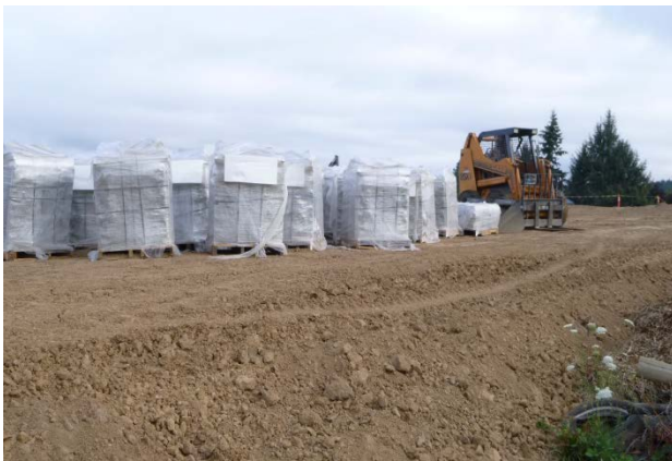
Retaining wall materials
