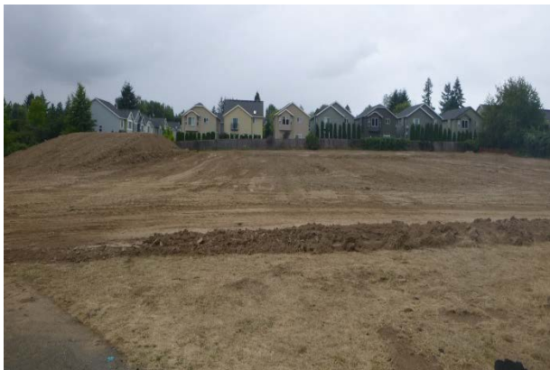
Site grading - looking south
