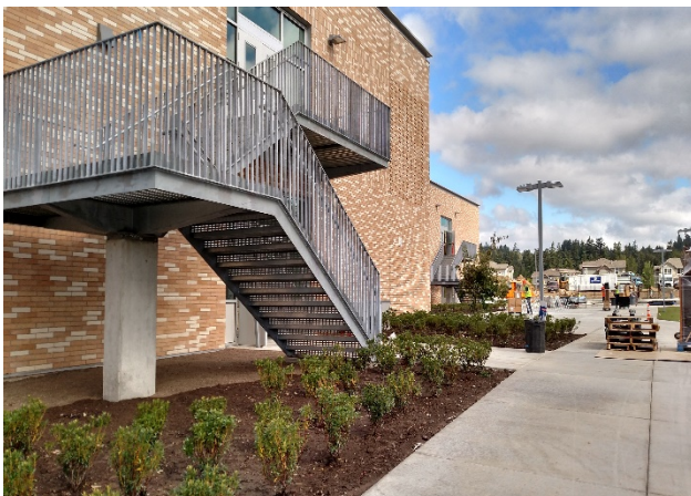
Outside exit of central classroom wing
