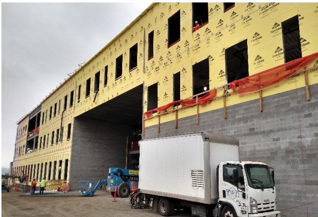
Classroom wing - looking south
