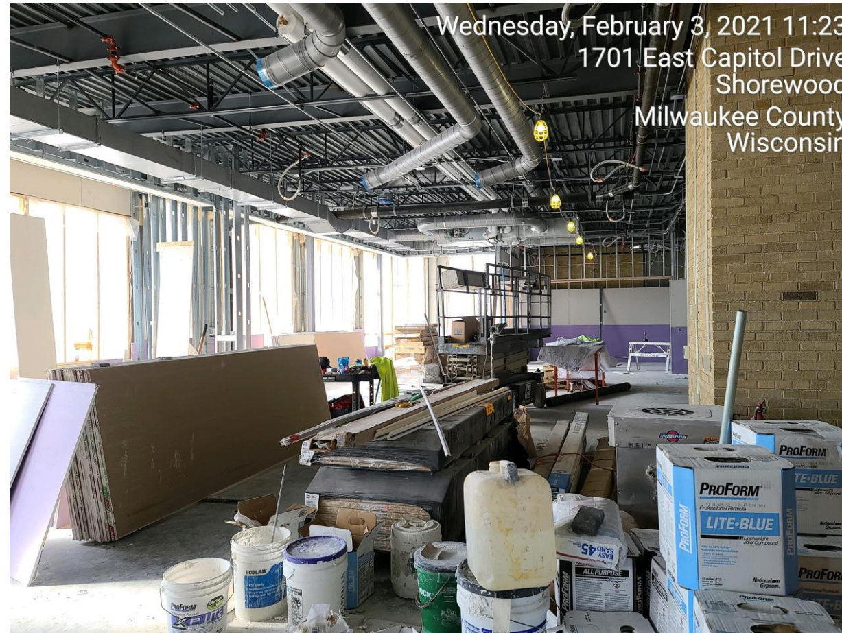
View from inside new addition on the 2 nd floor
