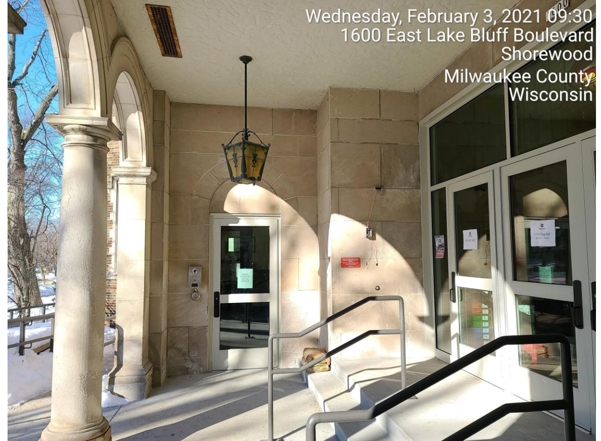
New secure and ADA entrance (exterior)
