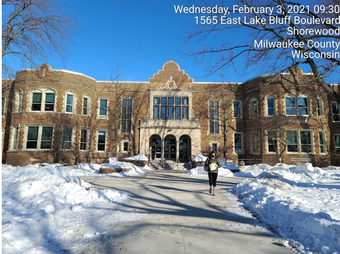
New Window installation is complete
