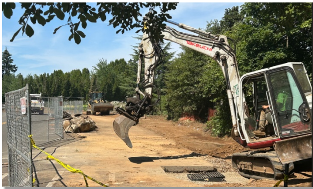
Loop Trail Progress! Left is the ADA Ramp to Green Lot, Right is Solving a Drainage Problem
