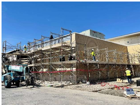
Brick Installation on Addition at Alumni Hall
