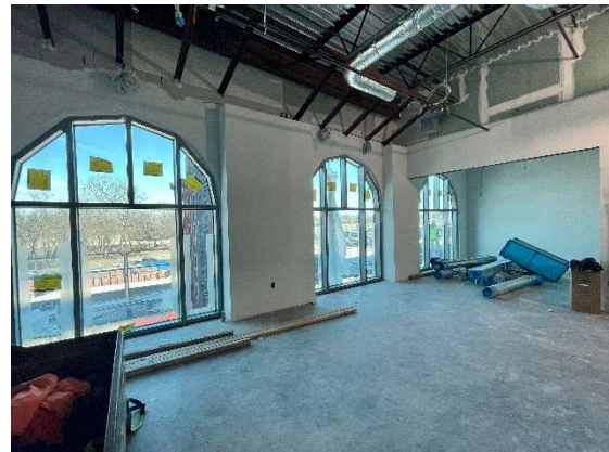
Vet Lounge on 2 nd Floor of Welcome Center
