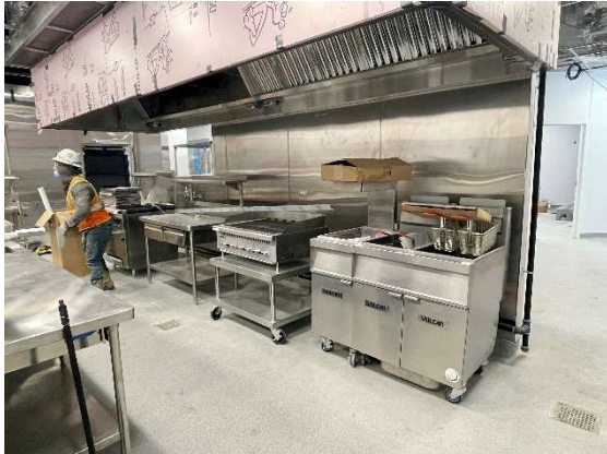
Kitchen Equipment Installed
