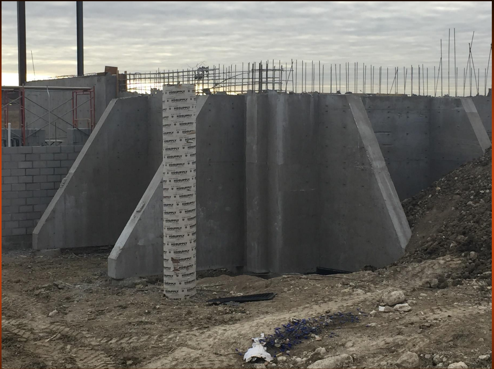
Elementary 5 Crawlspace Buttress Walls
