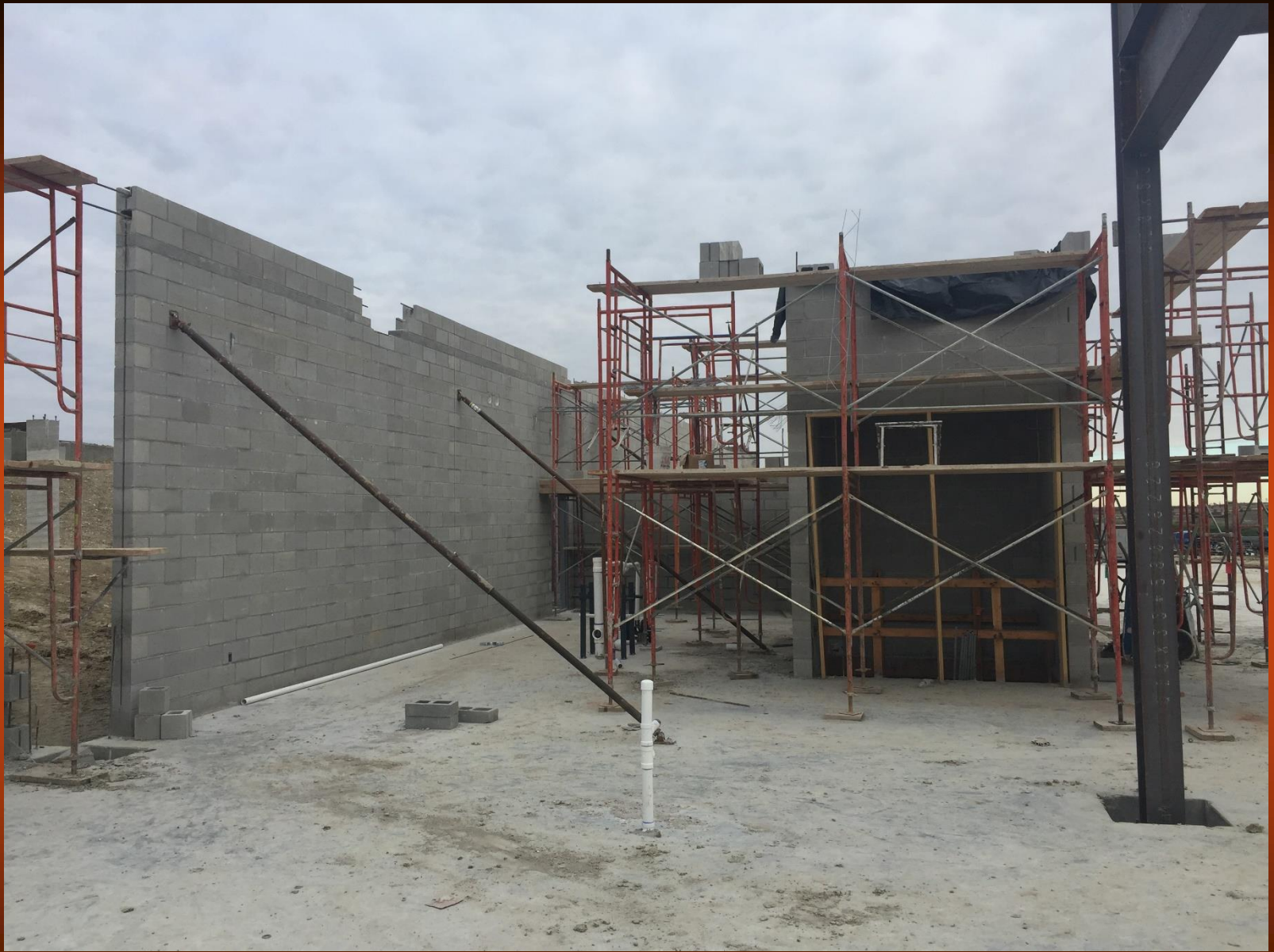
Elementary 5 CMU at Crawlspace Wall and Elevator Shaft
