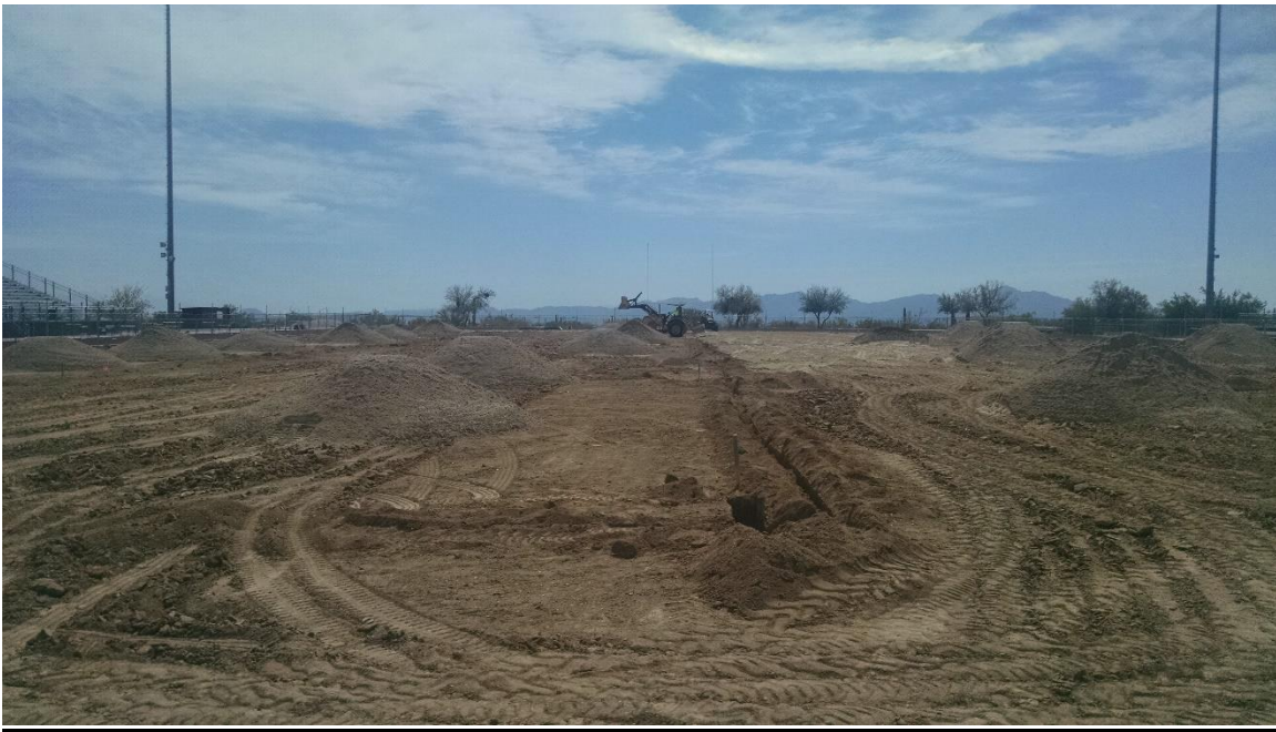
Football field under re-construction
