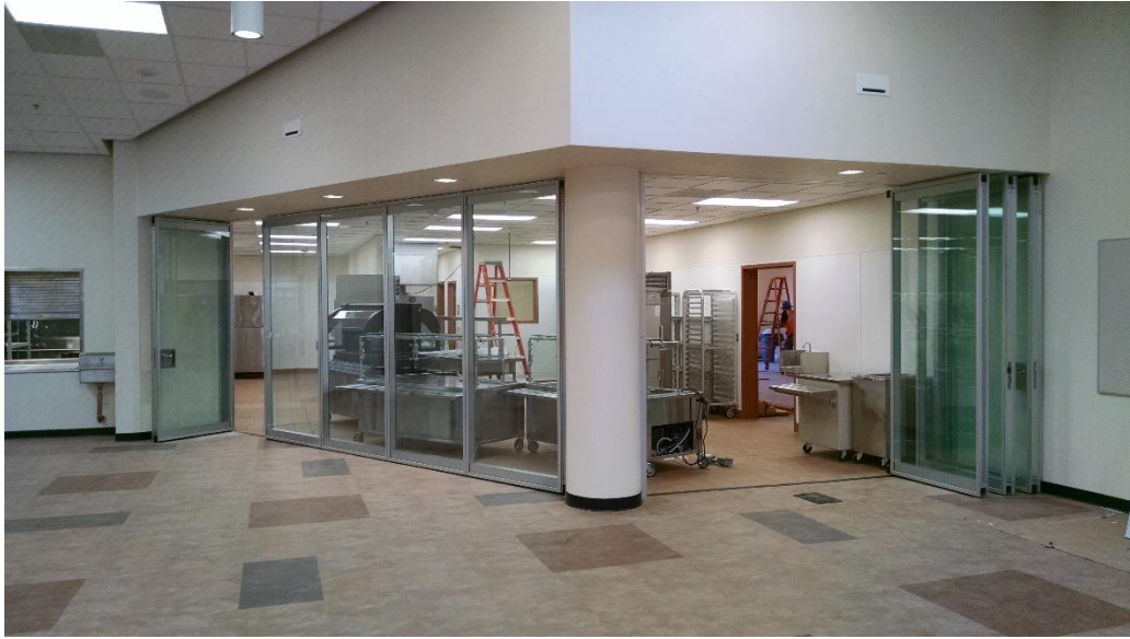
300 Building kitchen area
