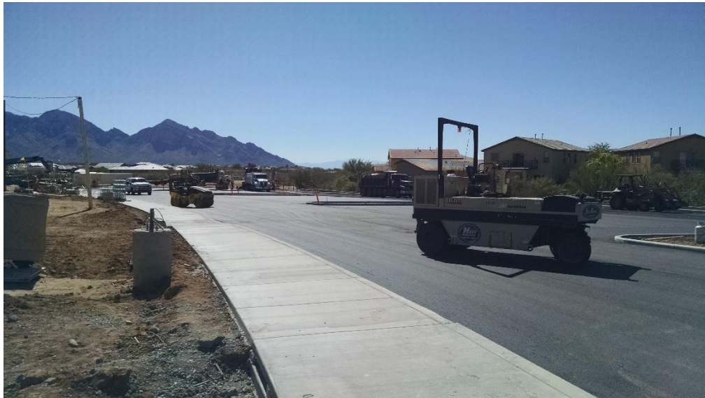
Parking Lot and Sidewalks on the West side of Campus
