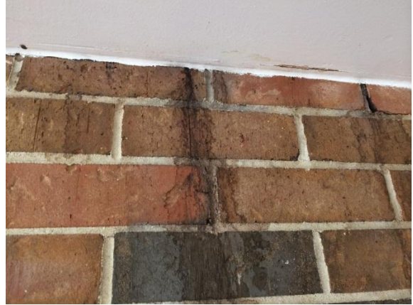
Photo 2: Vestibule Ceiling / Wall
