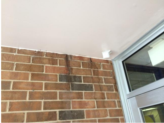
Photo 1: Vestibule Ceiling / Wall
