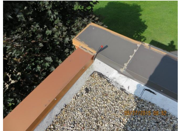
Photo 15: SE Roof Coping Intersection
