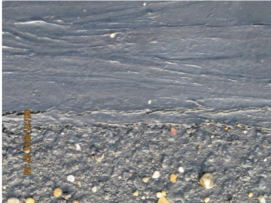
Photo 18: Roof Replacement Seam
