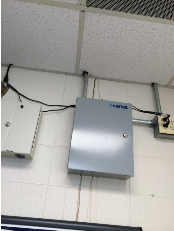
Photo 5: Wall – Secretary to Vestibule
