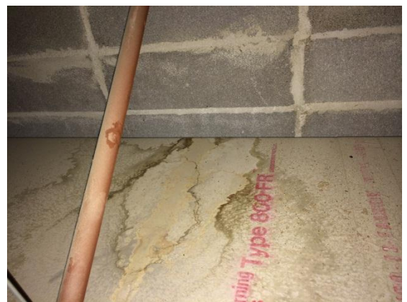
Photo 12: Room 118 Corridor Wall
