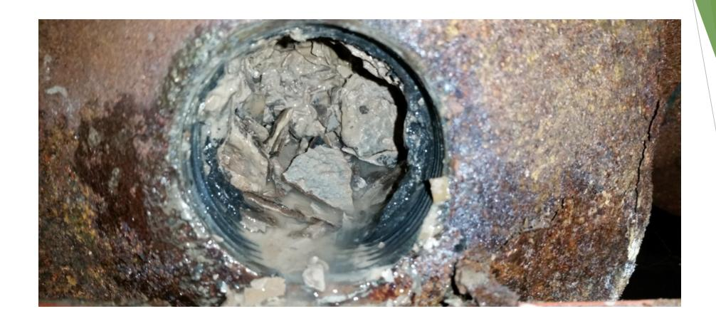
Sediment on water side port. We had to pound sediment out with a piece of conduit and a sledgehammer.
