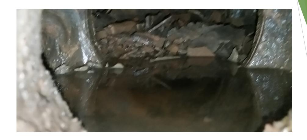
Sediment inside the boiler coming off the 4" drain line
