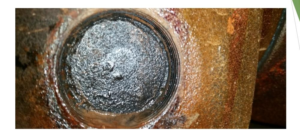
Water Side port clean outs corroded and loaded with scale.
