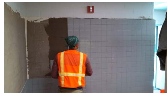
D Bldg. Restroom Renovation (setting tile)
