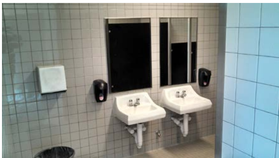
B Building Completed Restrooms
