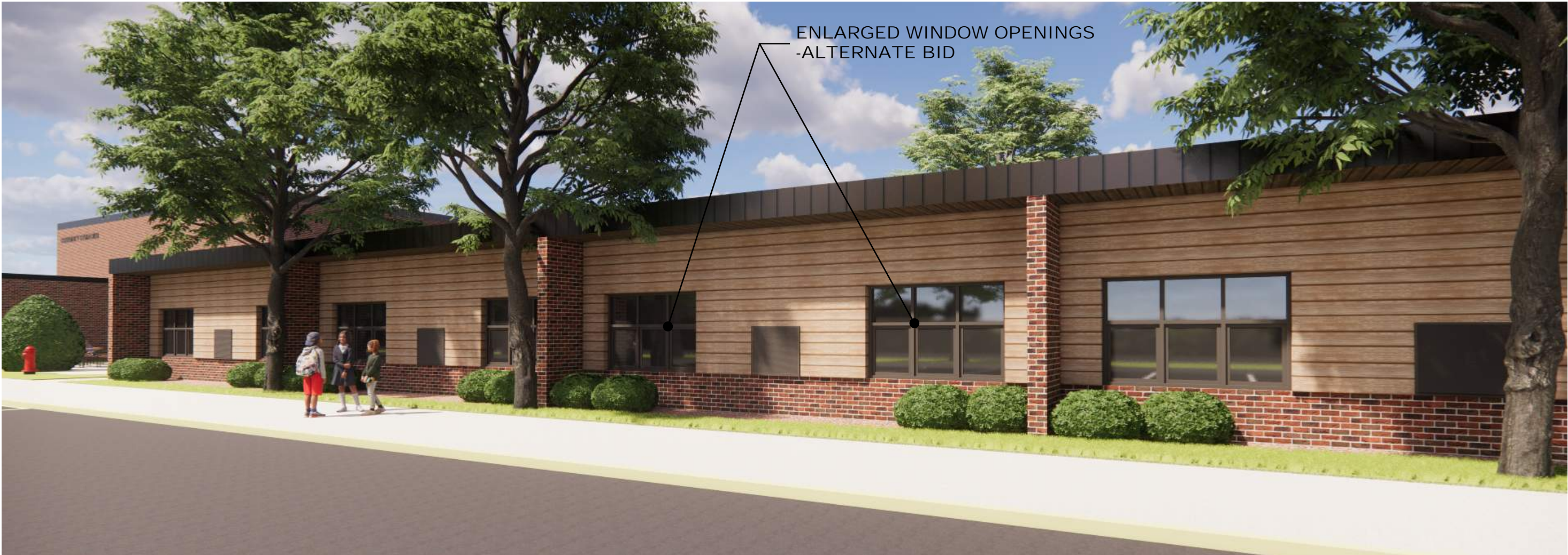
NEW PANELING REPLACES OLD PANELING ON SCHOOL ELEVATION, NEW WINDOW TYPE, AND ENLARGED WINDOW FENESTRATION
