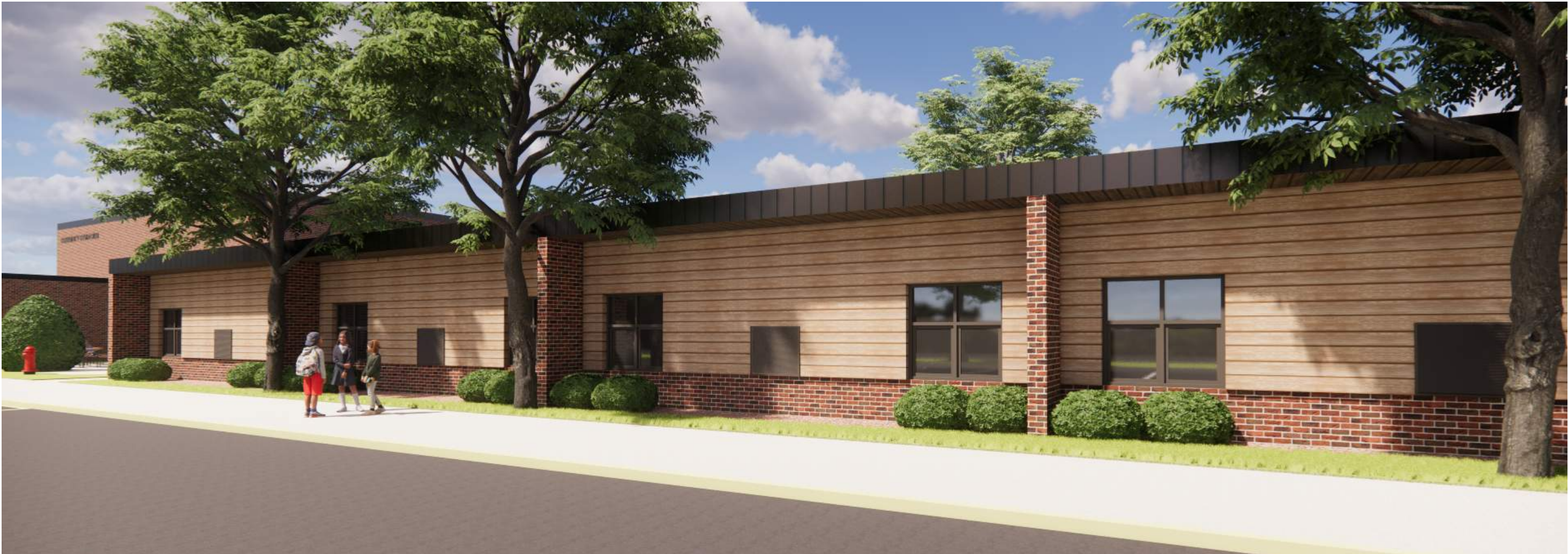
NEW PANELING REPLACES OLD PANELING ON SCHOOL ELEVATION AND NEW WINDOW TYPE
