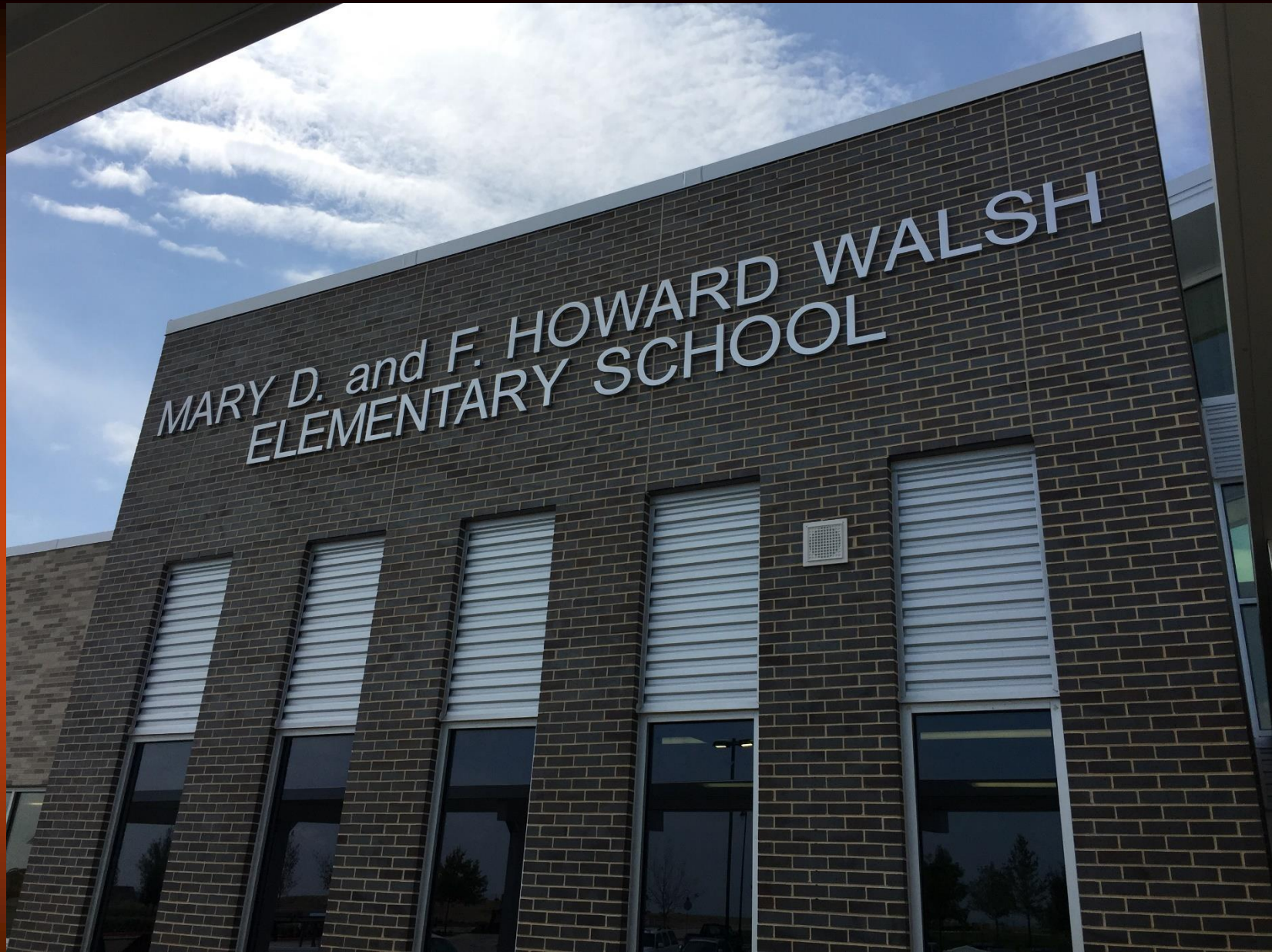
Walsh Elementary Building Letters
