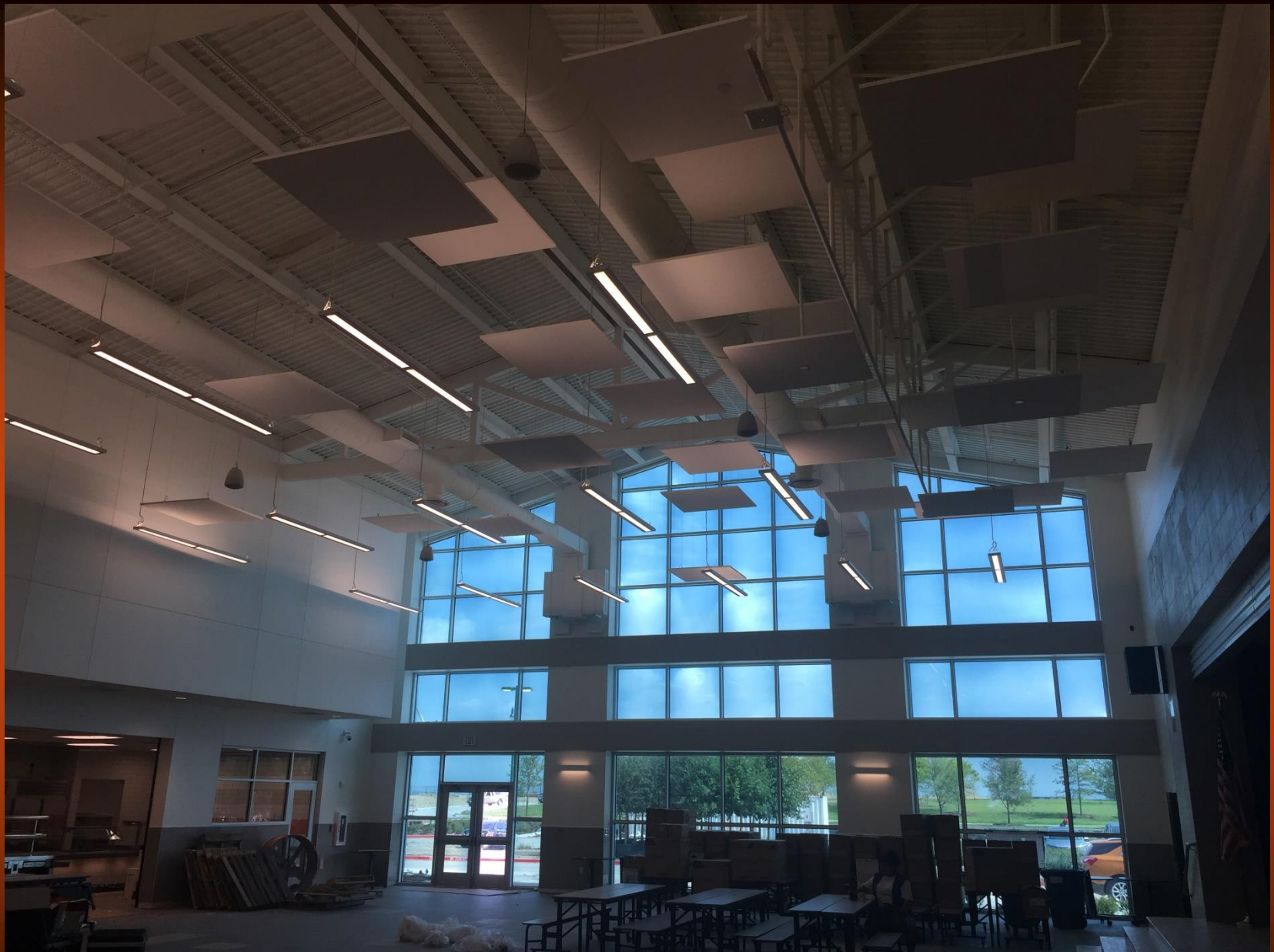
Walsh Elementary Cafeteria and Ceiling
