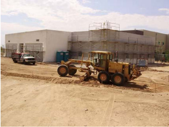
Bus lane excavation
