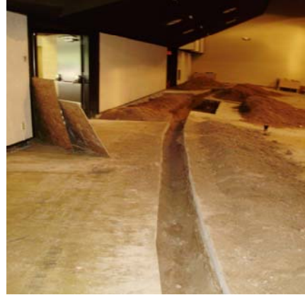
New electrical trench in auditorium floor
