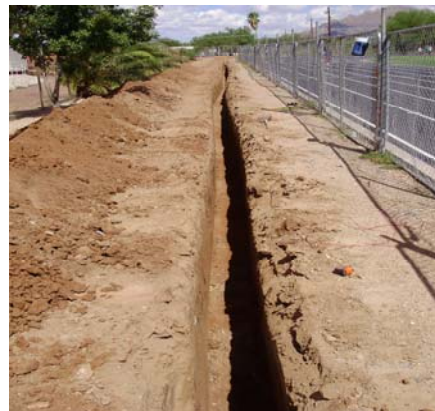
New mainline trench
