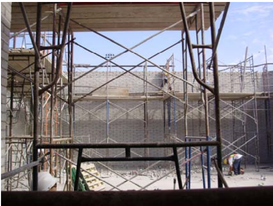
New Kitchen exterior walls (interior view)
