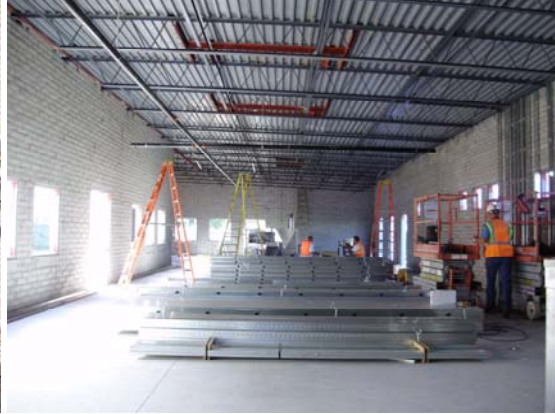
New classroom roof decking
