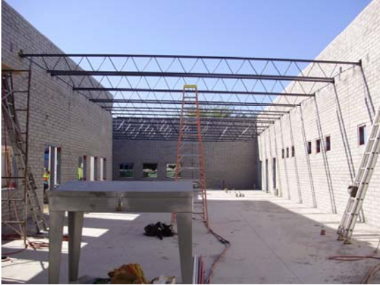
New classroom walls and roof framing
