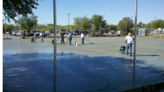
Concrete Pad Finishing
