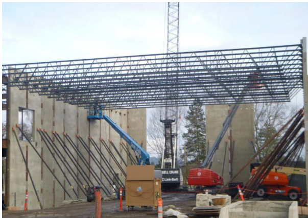
Truss installation
