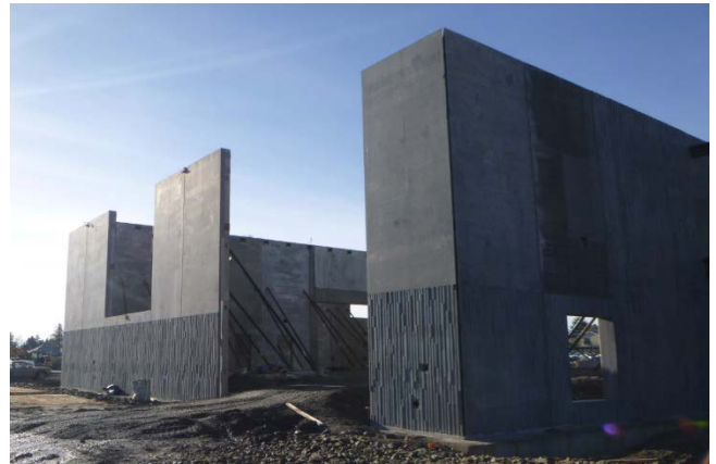
Precast panel installation
