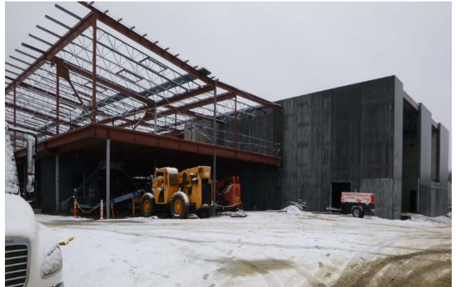
Precast panels and structural steel
