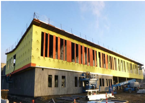
Exterior sheathing and vapor barrier
