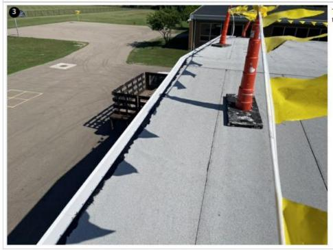
The gutter and drip edge are complete on the southern slope of the main roof section.
