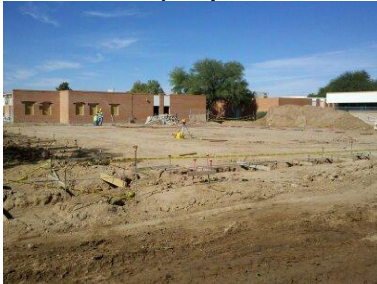
Pad and Footer Trenches for New Classroom Building
