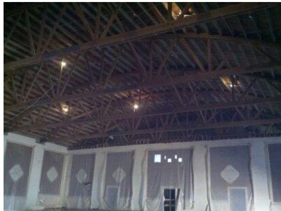
Exposed Bow String Trusses
