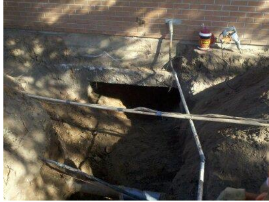
Tele-data Trench for Feed Into Library IDF
