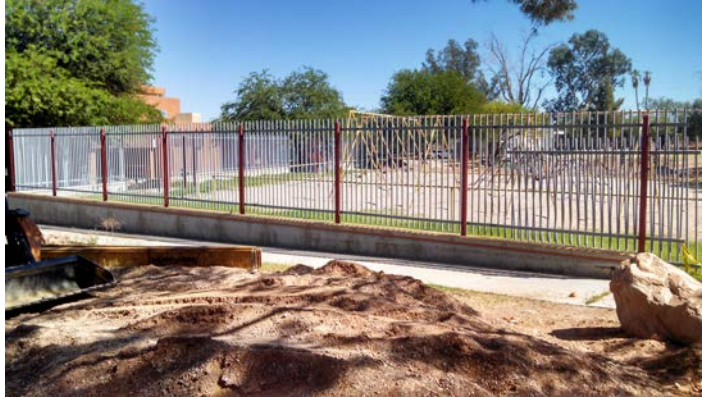
New Security Fence Installation
