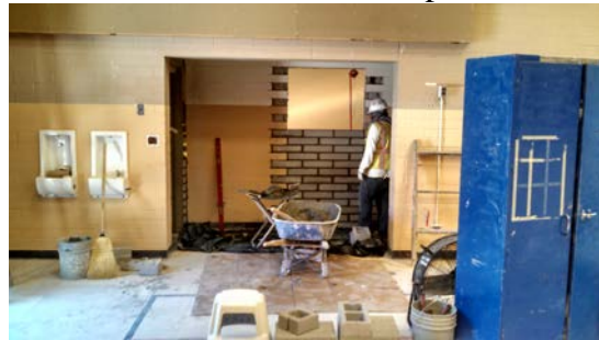
Restroom Renovations (in MPR and Admin)
