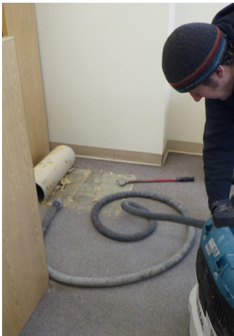
Floor Slab Testing
