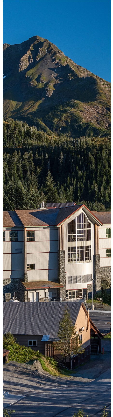
Cordova Center, MRV Architects
