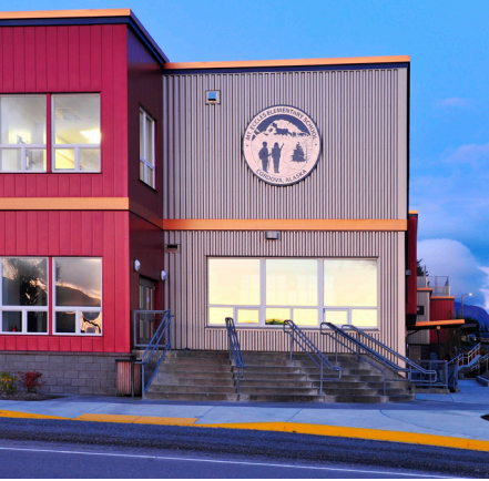
Mt. Eccles Elementary, Cordova, MRV Architects
