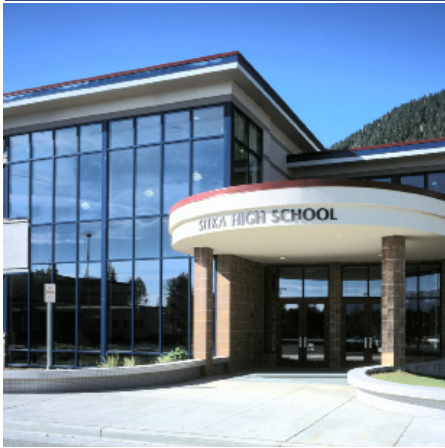
Sitka High School Renovation, MRV Architects
