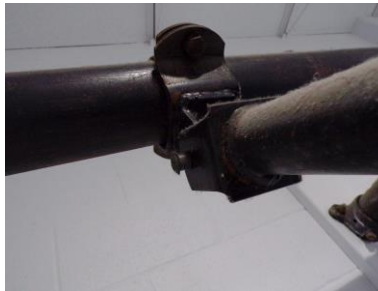
Pivot bolt need replacement
