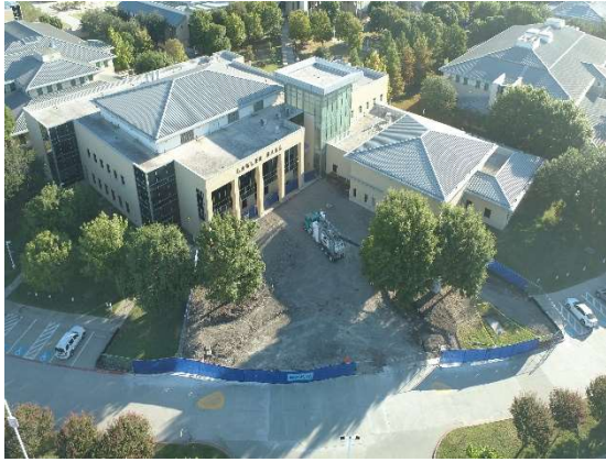
Lawler Hall Aerial for September '21
