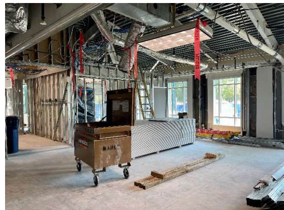
Interior Renovations Founders Hall
