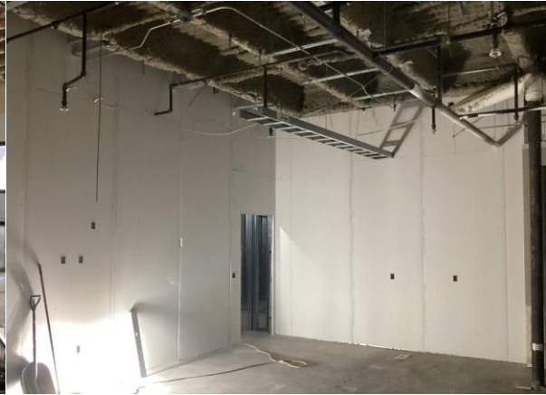
Drywall Installation
