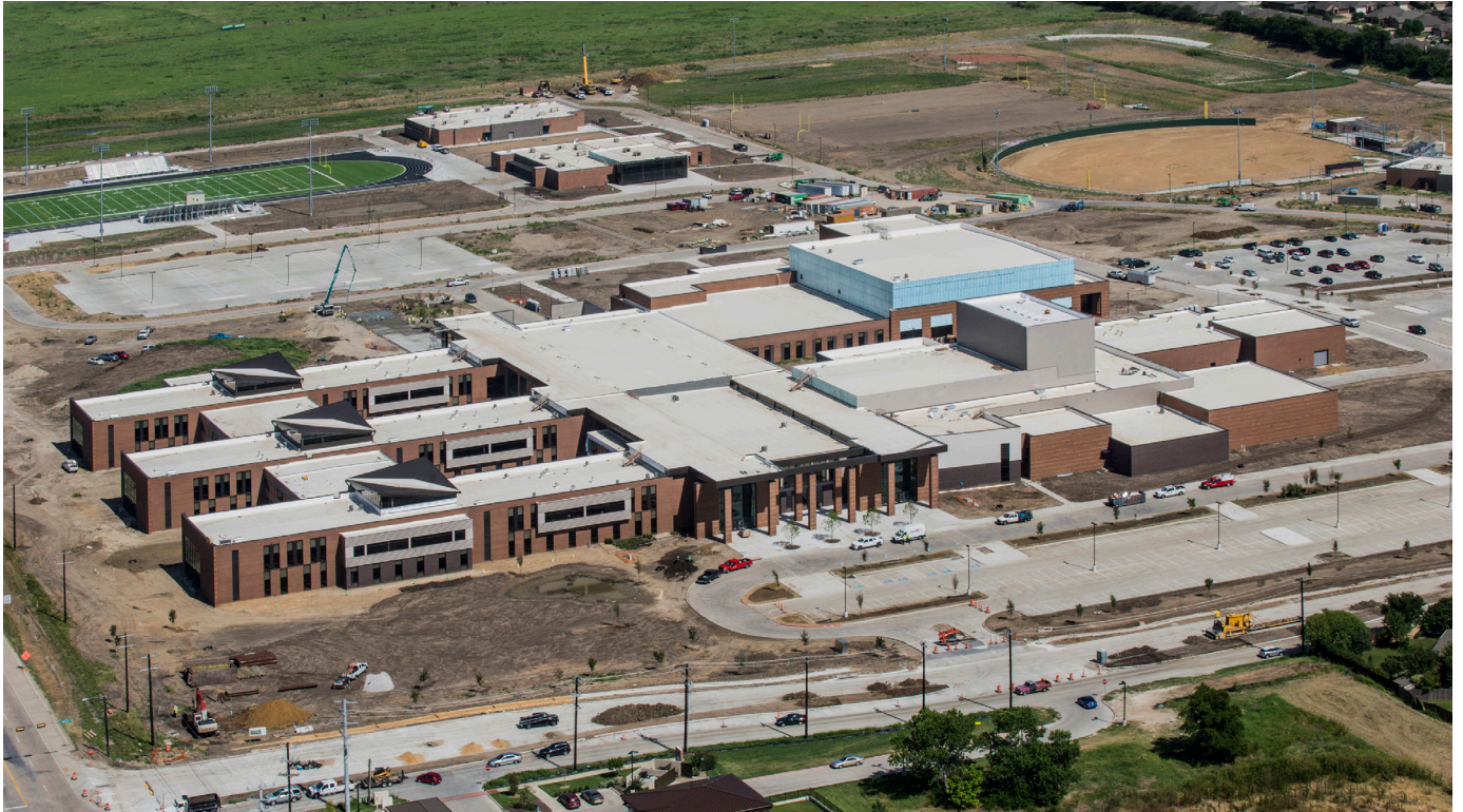
Aerial of main building
