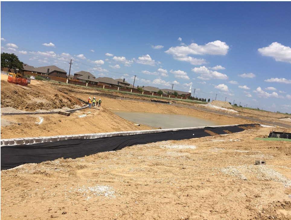
Pond retaining wall is being constructed.
