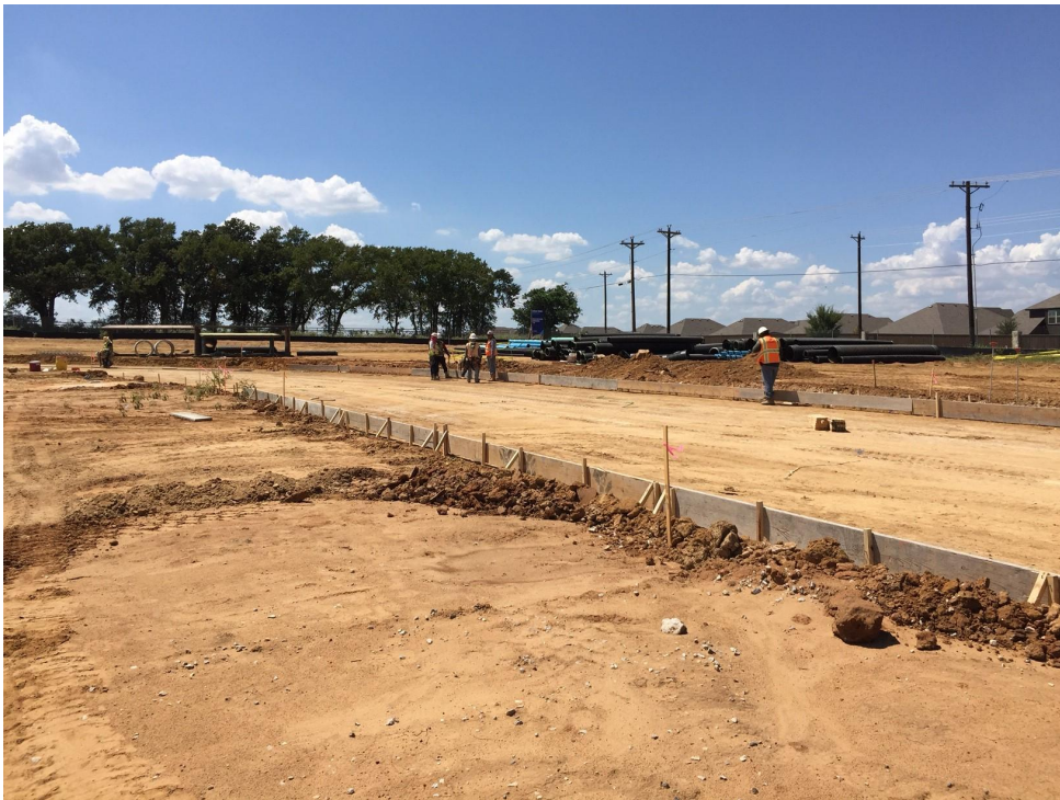
Fire lane paving is in progress.
