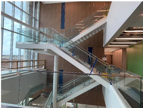
Glass Handrail Installed at Staircase
