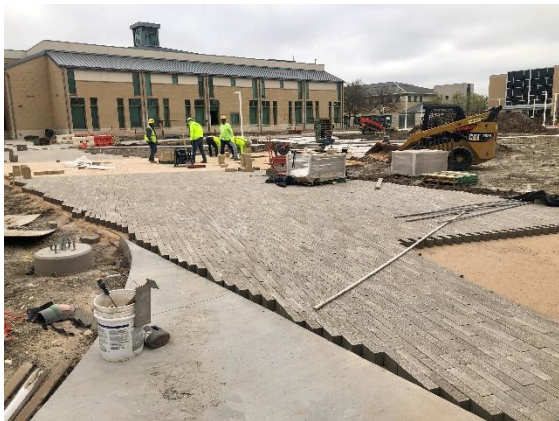
Quad Area, South of Building
