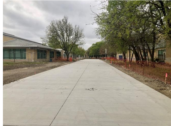
Fire Lane Poured, North to South View
