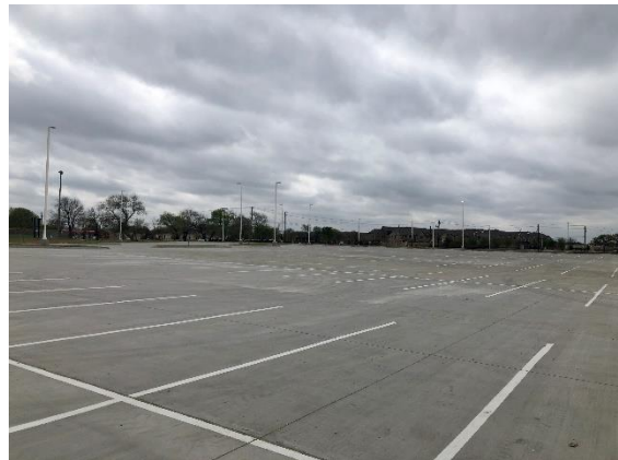
North View of Parking Lot
