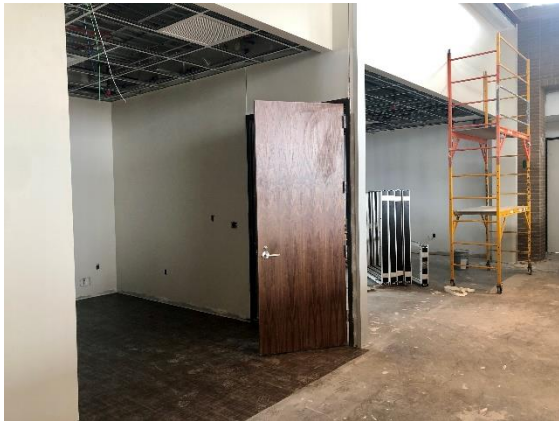
Dean's Suite on 3 rd Floor, North Side of Building
