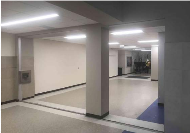
Area D 1st Floor Bldg. Connection
