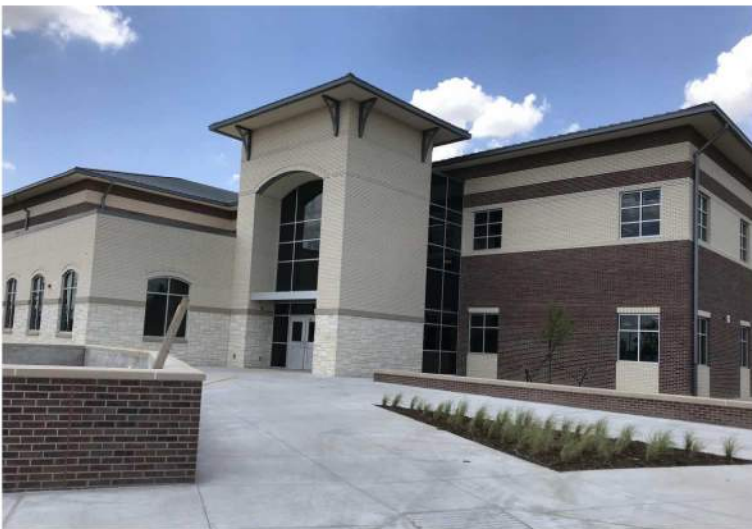
Area E Front Entry Vestibule
