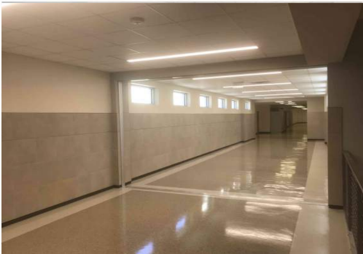
Area D 2nd Floor Bldg. Connection
