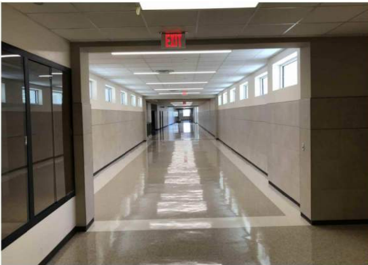
Area D 2nd Floor Bldg. Connection
