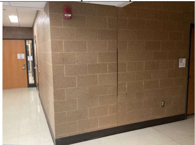
Missing sealant
